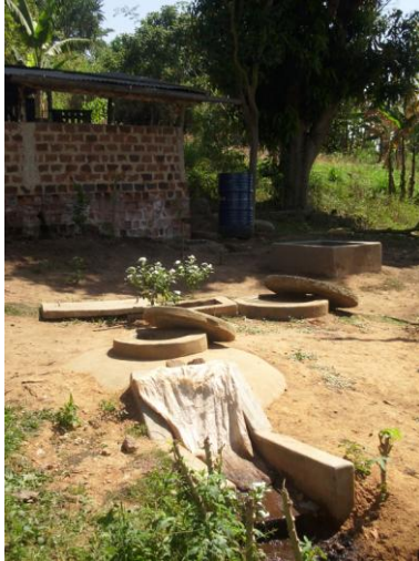
Figure 3. Small fixed dome digester at a pig farm in Buwambo
