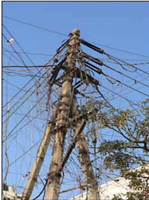
Figure 1: Illegally Tapping into the Power Line
