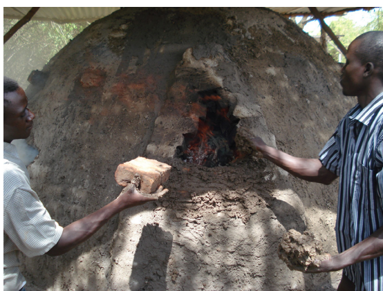
Figure 4.3: Sealing the doorway of a half orange kiln (Nellie Oduor, KEFRI)
