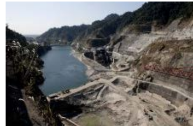
Lower Subansiri dam and power station in Arunachal Pradesh, Northeast India/ Tania Ghosh - Panos London
