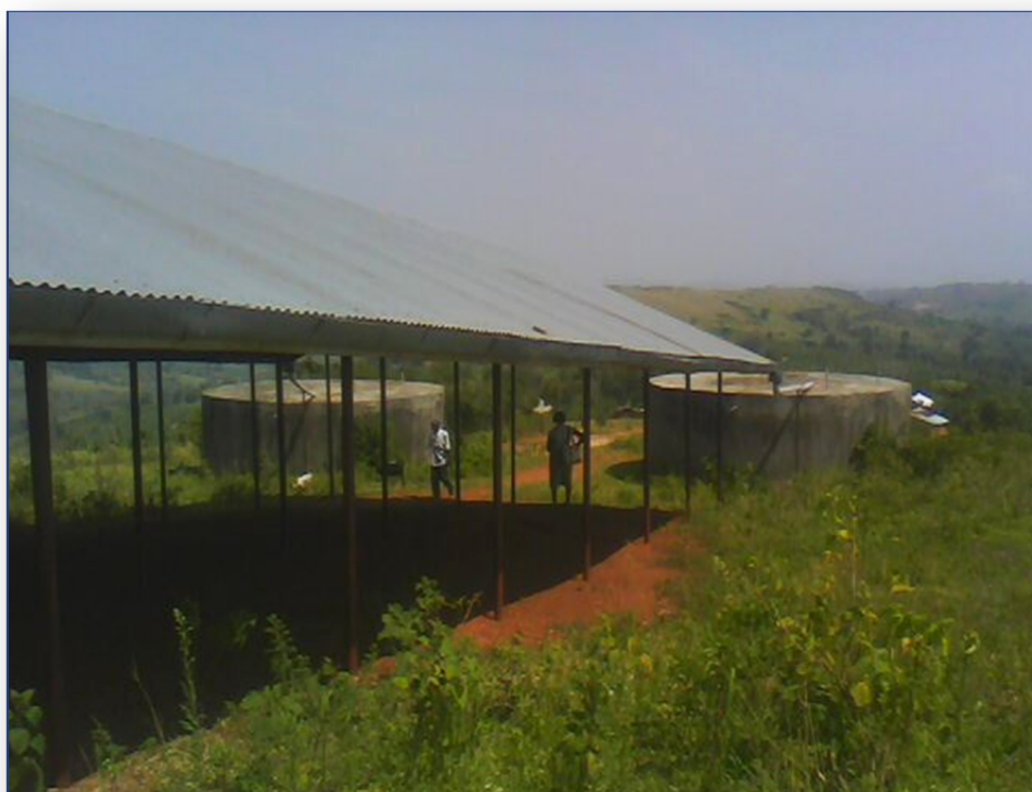
A ferro-cemented tank built by an NGO in Dwaniro sub-county, Rakai district: maintenance becomes a problem when communities take over such facilities
