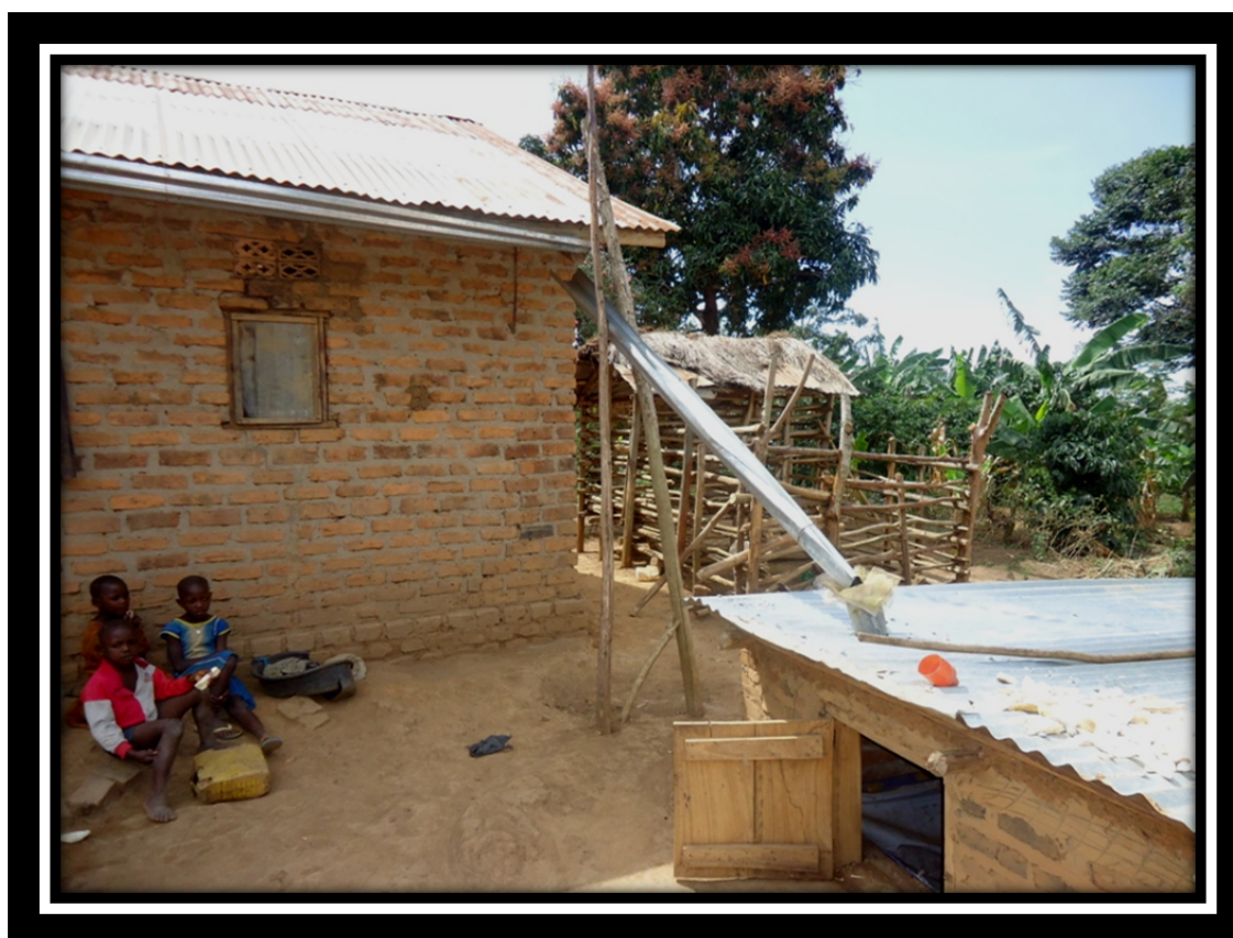
An underground water harvesting tank in Dwaniro sub-county, Rakai district
