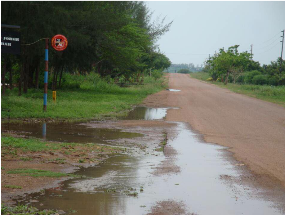
Low lying area with poor drainage
