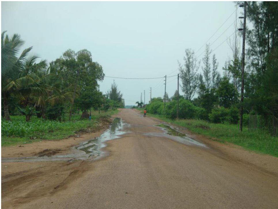
Low lying area with poor surface drainage
