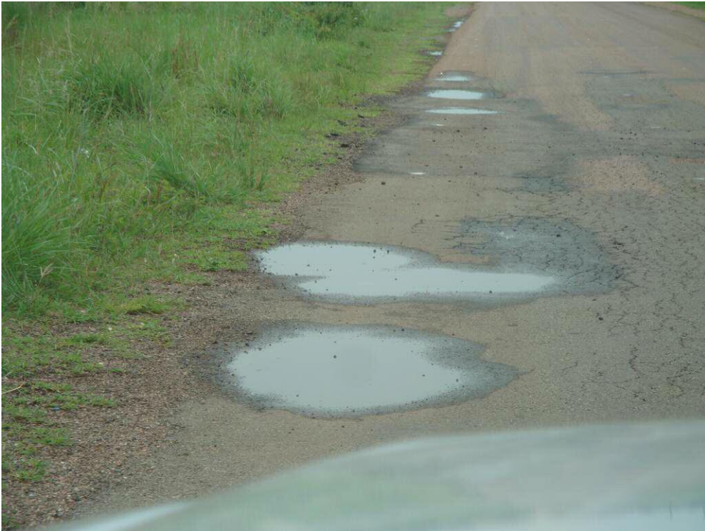
Deformation on wheel track probably due to poor drainage
