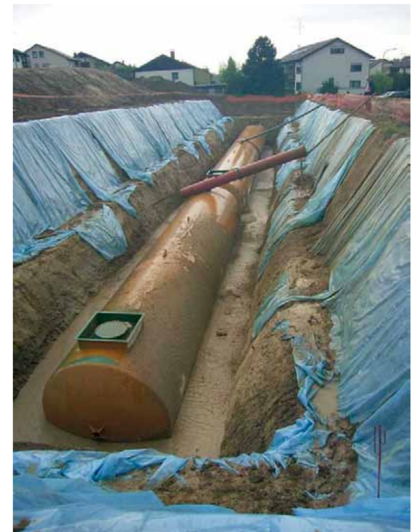
Rainwater storage tank :
