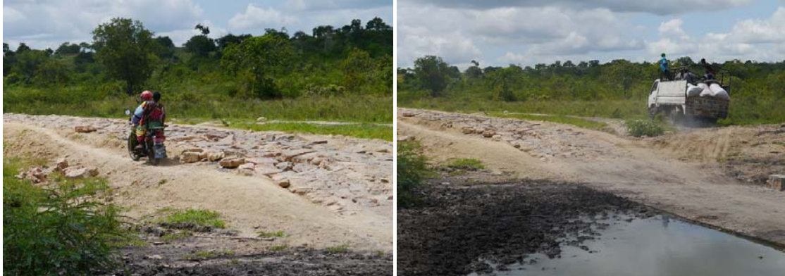
Failed road section of packed stone. Motorcycles now drive on the shoulder while trucks take a bypass through the bush
