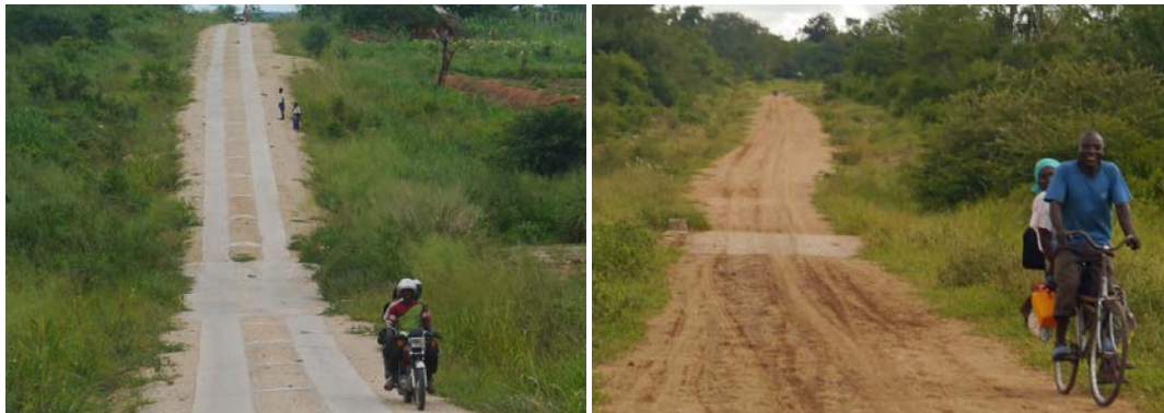
Left: Motorcycle taxi on experimental section with concrete strips. Right: Bicycle and passenger.
