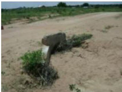
Nala – Veyula road: LHS – un de-silted culvert (Ch.3+600), Centre - vegetation control not done (Ch. 25+200) and RHS – point requiring drainage structure (Ch. 26+600)
