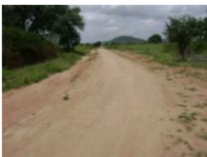
Mbabane – Chizomoche road: Section of road that has been improved and is being maintained
