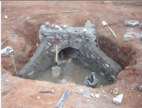
9: Construction of masonry headwall and wingwall
