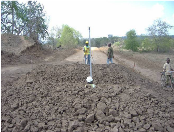
2: Setting level of culvert
