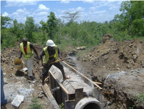
11: Curing the concrete
