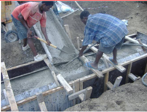
7: Compacting concrete
