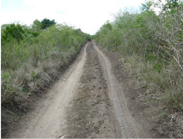
1: Before construction Chainage: 6+200 km
