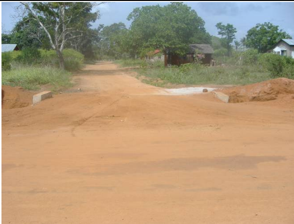
12: Backfilling of culvert using in-situ material
