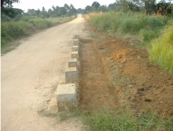
11: Excavation of gabion mattress
