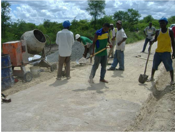
10: Spreading thin layer of sand to level base Date: 07/11/2011
