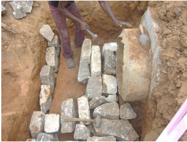
8: Construction of apron
