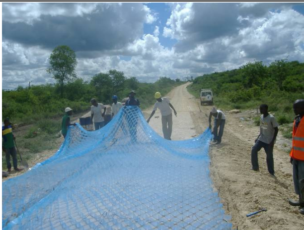
12: Laying out of geocells Date: 07/11/2011
