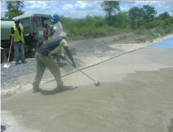
17: Brush stroke finish to concrete Date: 08/11/2011
