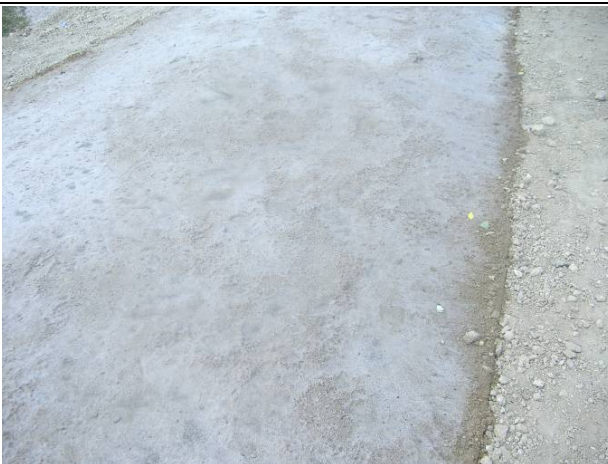
18: Curing of concrete with sand Date: 09/11/2011
