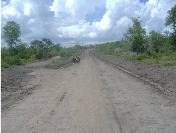
2: After heavy grading and compaction of the roadbed Chainage: 6+080 km Date: 29/12/2010
