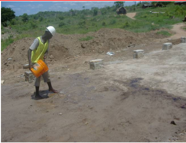
10: Curing the concrete
