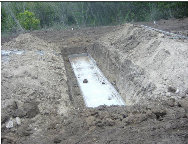
3: Cast concrete bed
