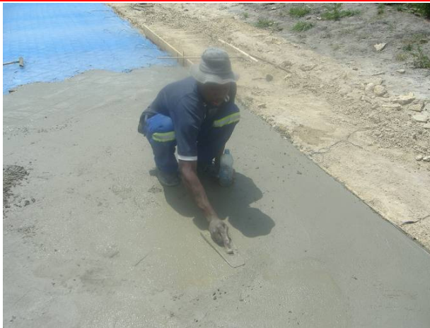
16: Smoothing concrete finish Date: 08/06/2011
