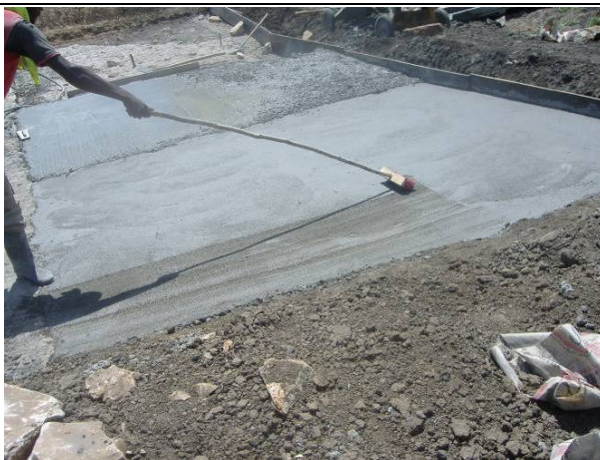
9: Brush stroke finish the concrete
