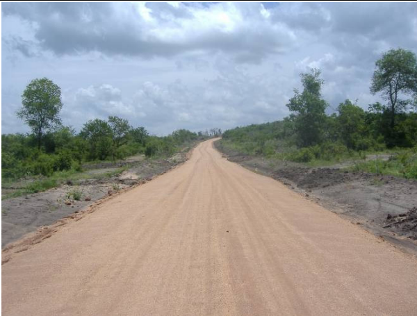
3: After spreading and compaction of 150mm of G7 improved subgrade layer Chainage: 6+080 km Date: 08/03/2011
