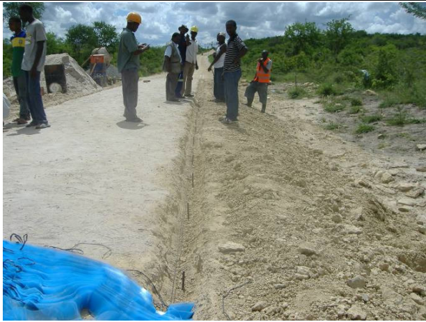
11: Setting out pegs to secure geocells Date: 07/11/2011
