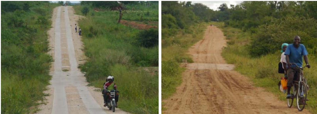
Left: Motorcycle taxi on experimental section with concrete strips. Right: Bicycle and passenger.
