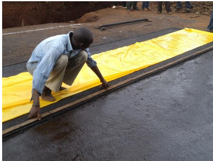
Photo 3-29: allowance for the construction of the adjacent strip by placing 6mm flat bar on top of the compacted asphalt (NB; use of plastic cover to protect damaging the fresh layer surface)
