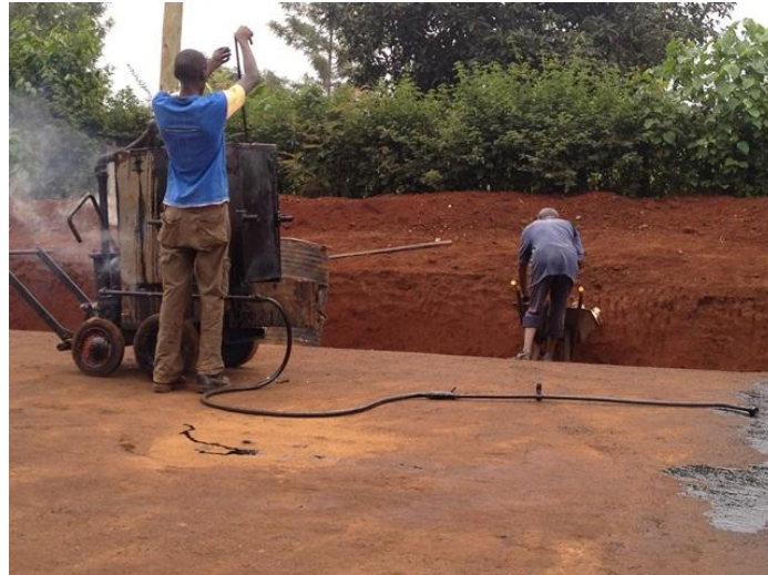
Photo 3-20: a thermometer fitted in the modified hand lance sprayer ensures the primer is applied at controlled temperature
