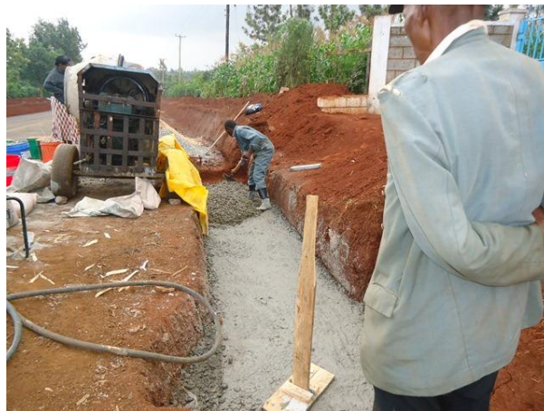
Photo 3-34: laying class 20/25 concrete mix on bed
