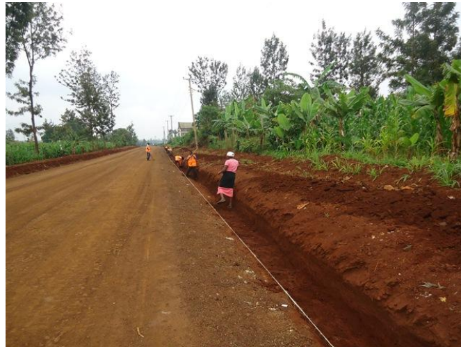
Photo 3-14: ditch formation in progress
