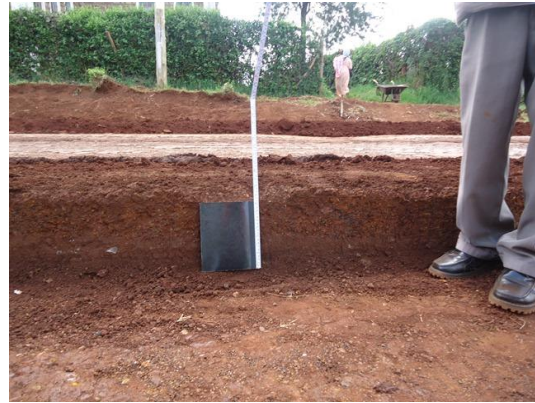
Photo 3-6: size of the 1st layer bench, 0+200LHS after compaction (approximately 120 mm)
