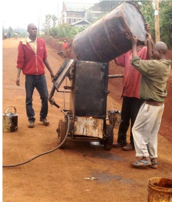
Photo 3-18: an improvised hand lance sprayer
