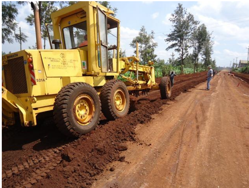
Photo 3-4: benching using a motor grader
