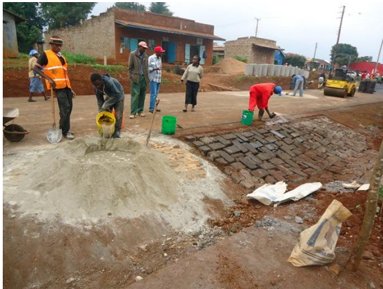
Photo 3-41: mortaring the drift
