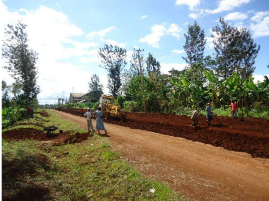
Photo 3-2: Top soil removal during stripping
