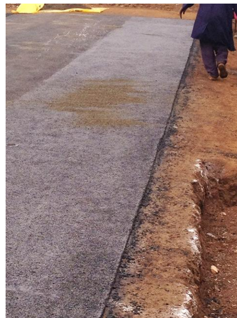
Photo 3-31: spreading of fresh cold mix to correct openings Photo 3-32: crusher dust used to seal joints
