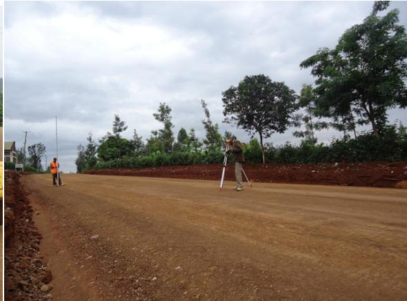
Photo 3-13: checking levels of the base
