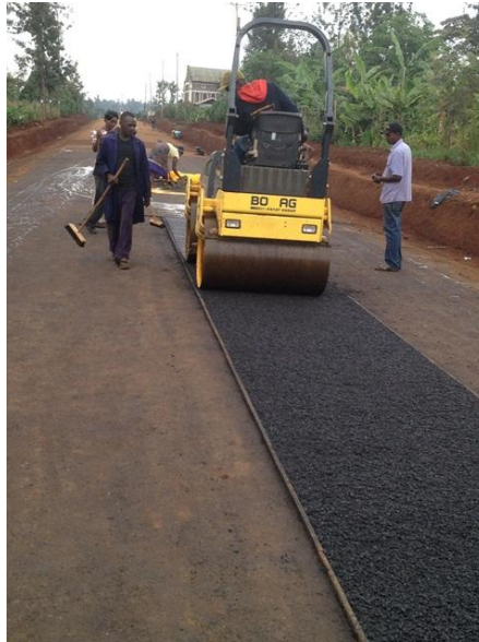
Photo 3-28: initial rolling of the cold mix asphalt layer with the roller in static mode
