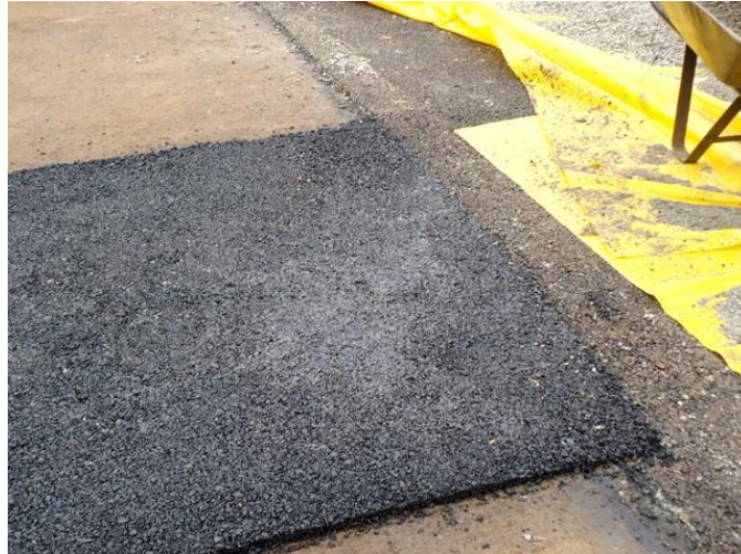
Photo 3-30: illustration of trimmed joints of a new layer adjacent to an old layer
