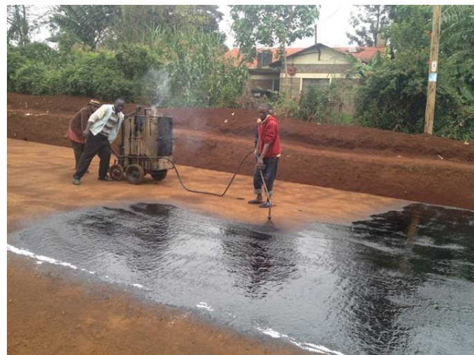
Photo 3-21; priming process in action
