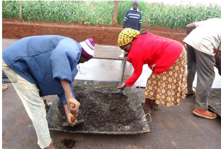
Photo 3-25: mixing of the cold mix asphalt using square nosed spades
