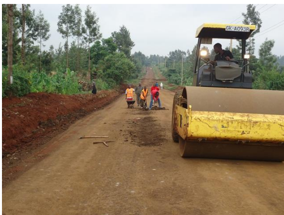
Photo 3-12: compacting the road base to refusal
