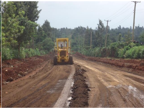
Photo 3-11: processing and grading of road base
