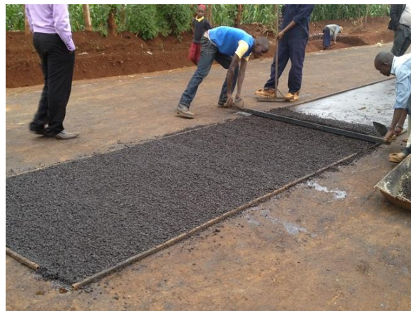
Photo 3-27: spreading and leveling the cold mix
