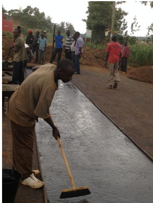
Photo 3-24: application of a dilute tack coat A-4
