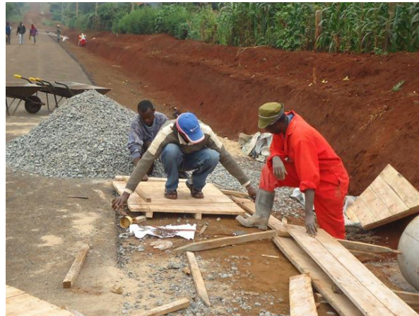
Photo 3-36: joining timber to form the false works
