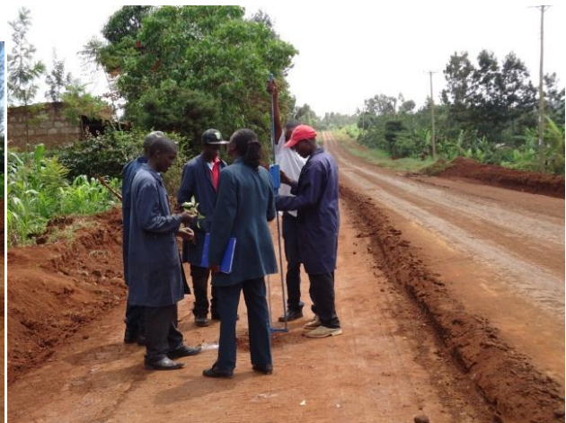
Photo 3-9: DCP test on the 1st layer bench
