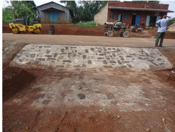
Photo 3-42: completed access drift
