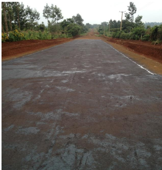
Photo 3-23: primed section ready for sealing
