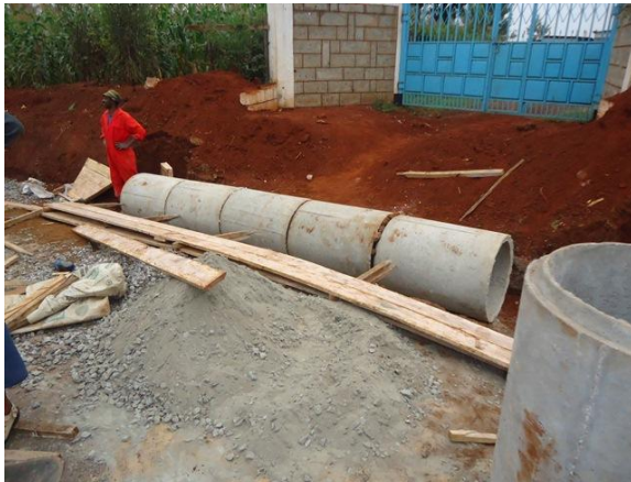
Photo 3-35: interlocking the culvert rings
