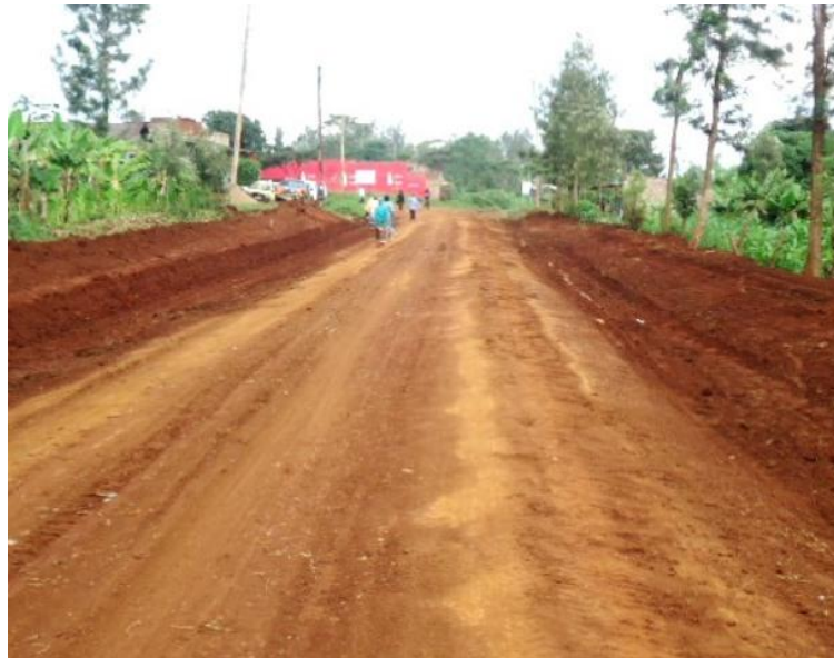
Photo 3-3: Section showing the process of stripping complete
