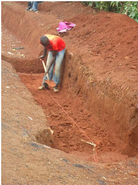
Photo 3-33: trench excavation for culvert bed
