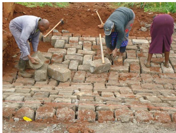
Photo 3-40: packing and interlocking the blocks
