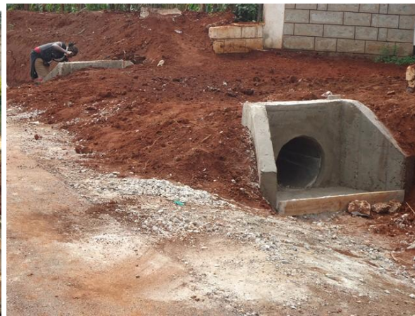
Photo 3-38: completed culvert-curing continues
