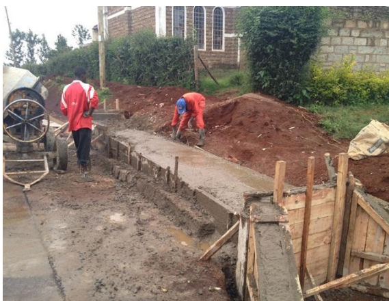
Photo 3-37: haunching of surround, head/wing walls
