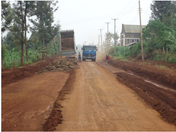
Photo 3-10: dumping gravel material for bench
