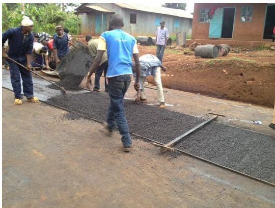
Photo 3-26: placing cold mix between guide rails
