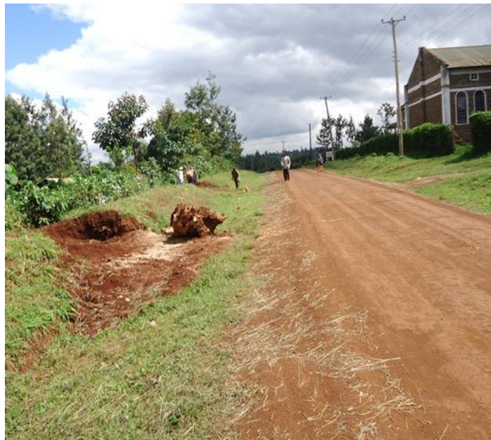
Photo 3-1: Stump removal during site clearing
