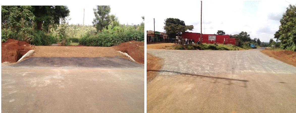
Photo 3-45: a view showing adjacent culverts with the finished road surface and the bell mouth
