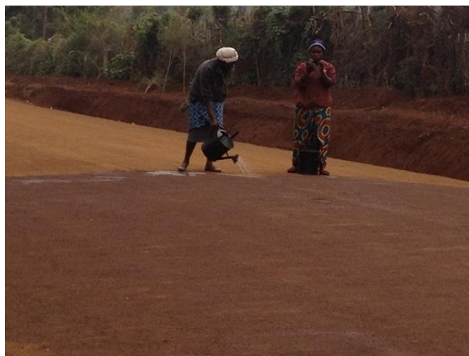
Photo 3-19: watering the broomed surface lightly using a free flow can
