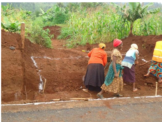
Photo 3-39: excavation of the drift level
