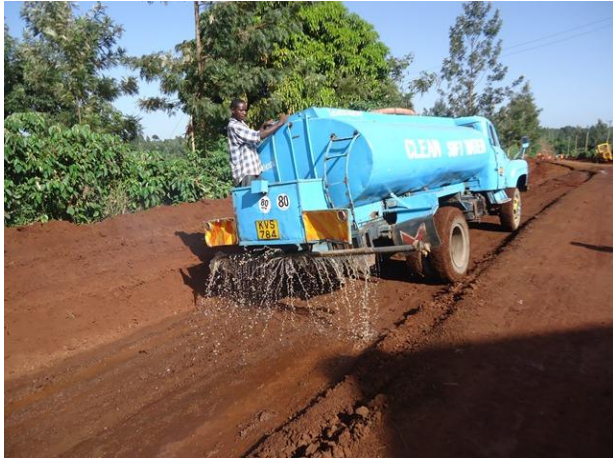
Photo 3-5: watering the bench during processing
