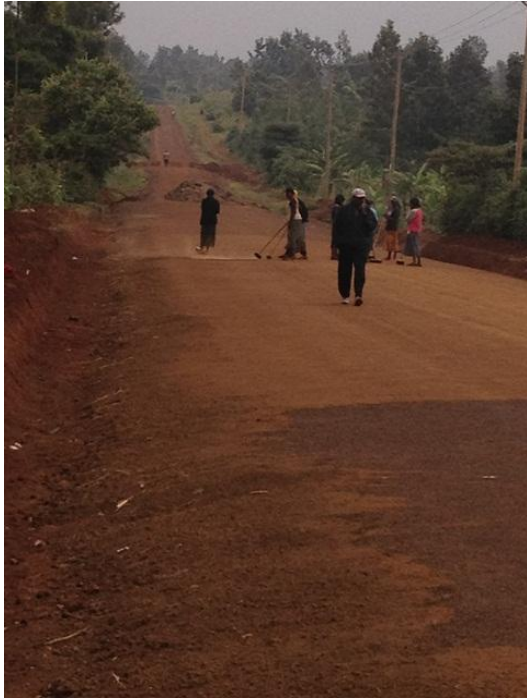
Photo 3-17: Brooming the compacted base surface
