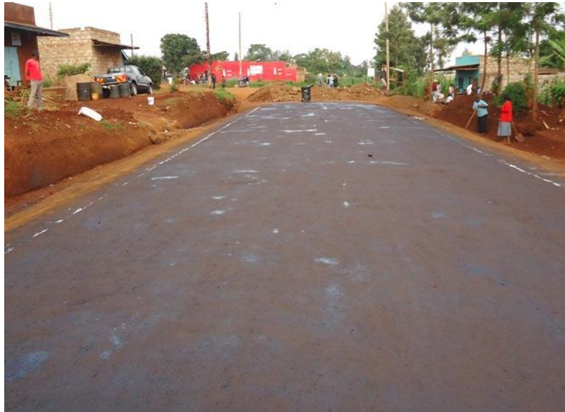
Photo 3-22: a section after 24hrs of priming. It was left further to dry for another 48hrs or more before surfacing for the MC 30 to penetrate fully
