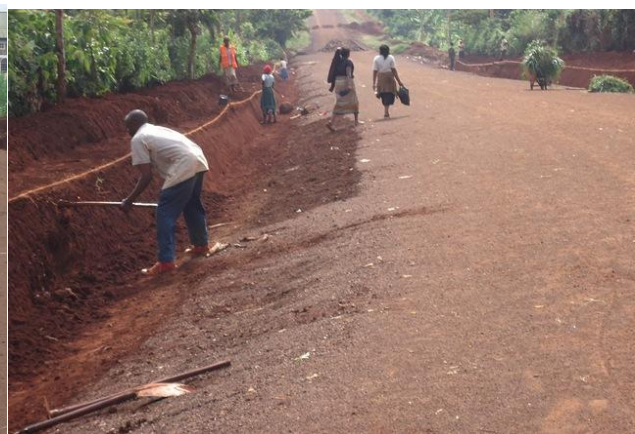
Photo 3-16: back slope formation and lining
