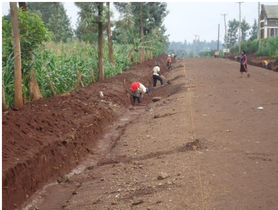
Photo 3-15: inner slope formation
