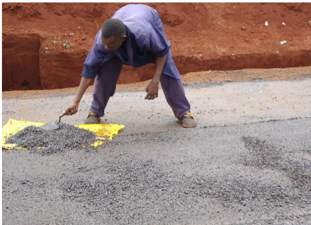
Photo 3-31: spreading of fresh cold mix to correct openings Photo 3-32: crusher dust used to seal joints
