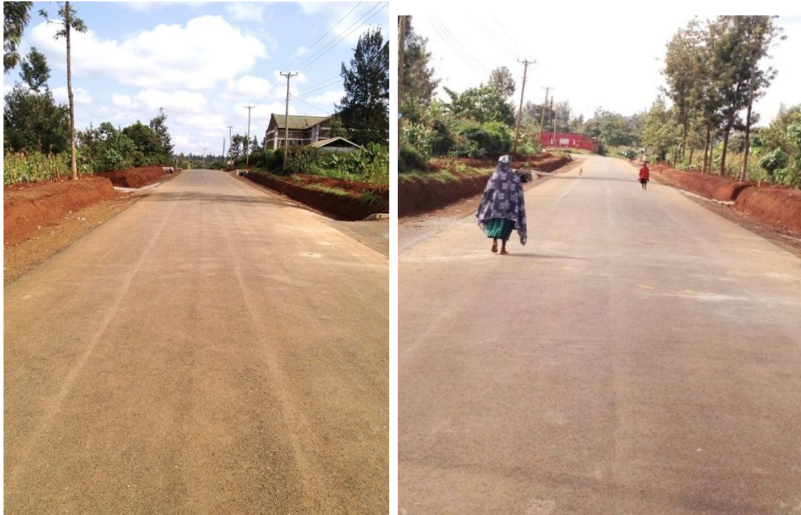
Photo 3-44: a view showing the finished road from Chainage 0+020 to 0+260 near the church junction
