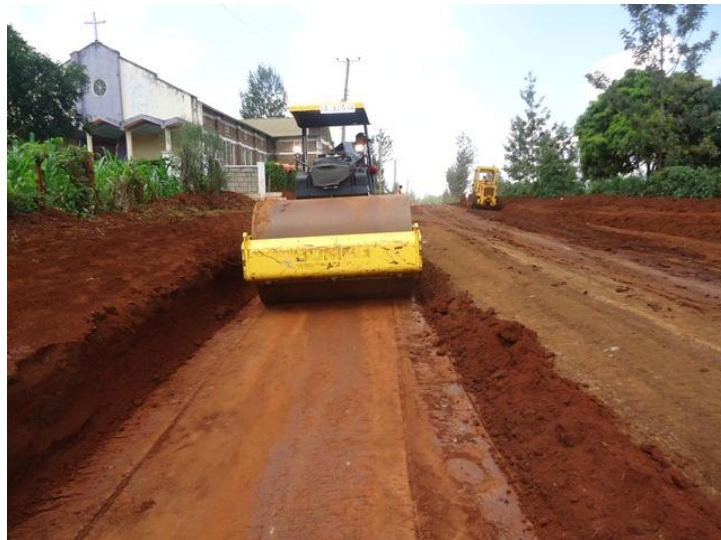
Photo 3-7: compaction on 1st layer RHS and processing on the LHS
