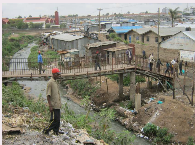
Hotspot Bridge in Mukuru
