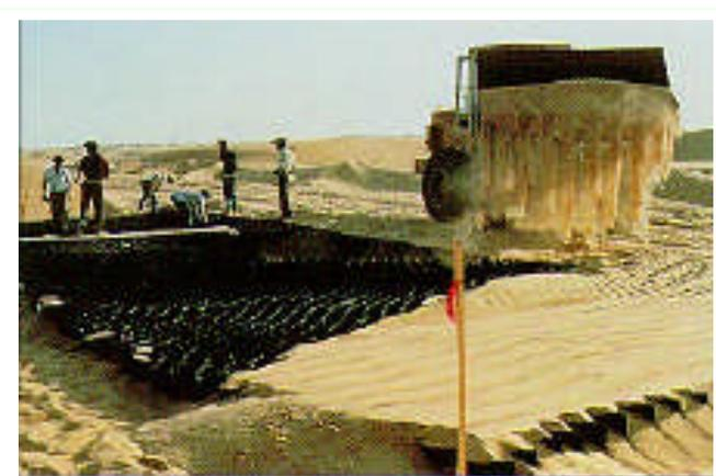
Sand filling of geocell by front end loader
