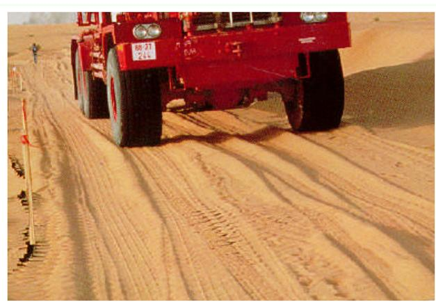
Use of sand-filled geocell by 40 tonne truck
