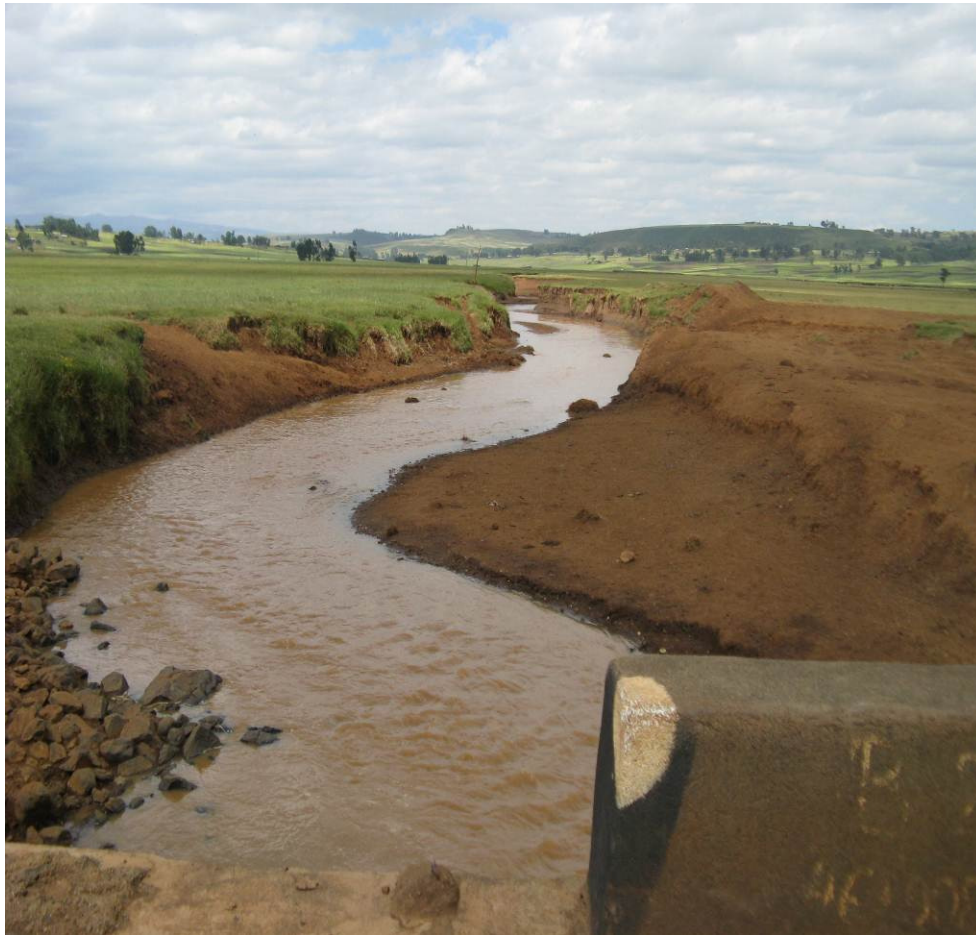
Figure 6.5 Meandering Channel on the Addis Ababa – Debre Markos Road
