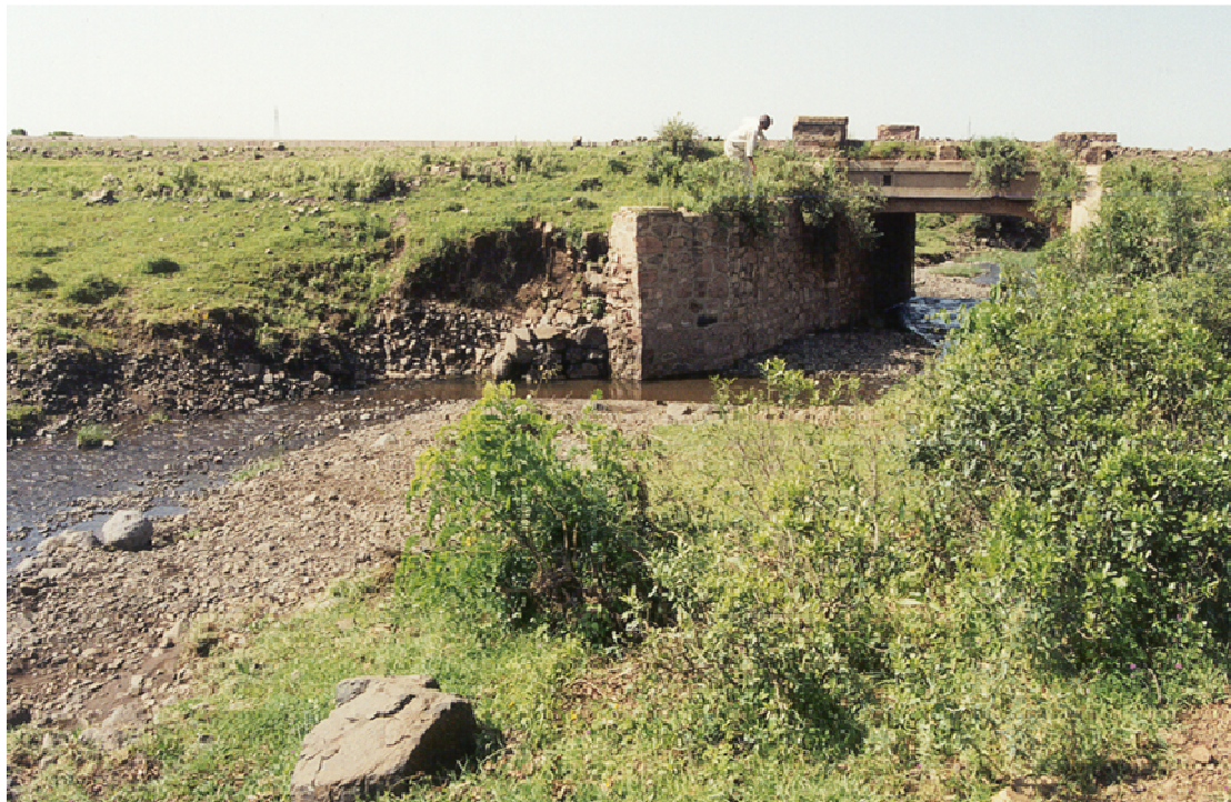
Figure 6.7 A Bridge where Meander Migration has Caused the Channel to Shift Laterally, Eroding the Adjacent Embankment, on the old Adwa-Adigrat Road
