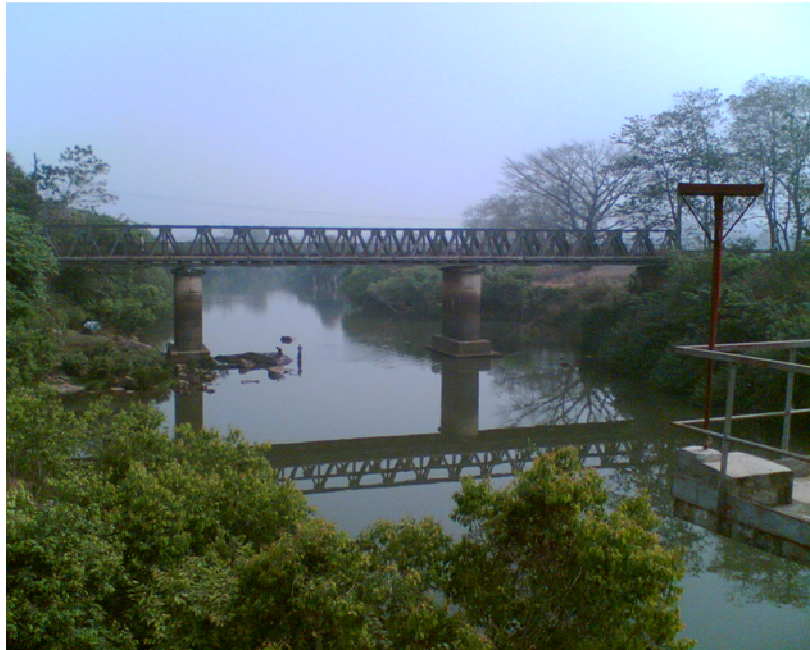
Photo 6.12 Bridge on a stable reach of channel in Guinea
