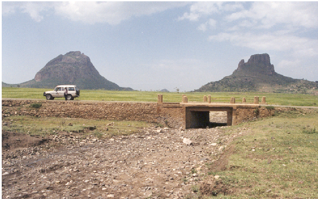
Figure 6.11 A simple culvert in essentially flat terrain
