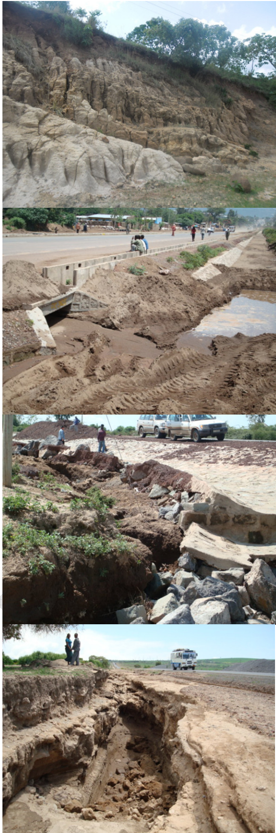
Figure 2 slope erosion, sedimentation of drainage structure and road side ditch (lined and unlined) erosion on dispersive soils (an example from a road project in the Rift Valley).
