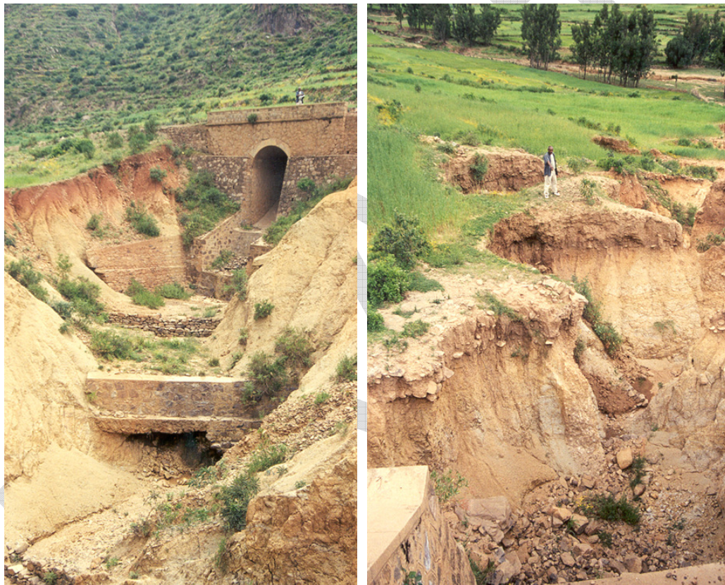
Figure 6.10 Gully Erosion on the Adwa-Adigrat Road
