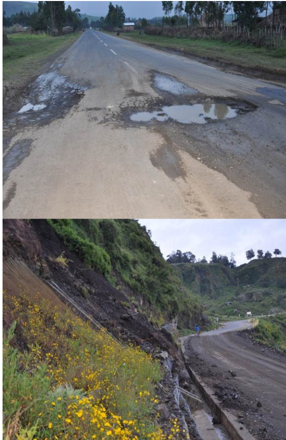
Figure 1 subgrade failure due to soil expansiveness resulting in road surface deformation and formation of potholes, and slope instability on colluvium with expansive (black cotton) soil matrix.
