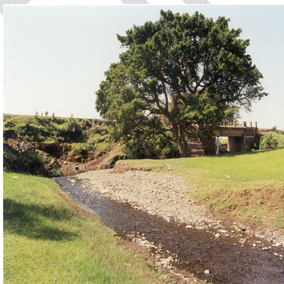
Figure 6.6 Meandering Channel on the Adwa-Adigrat Road
