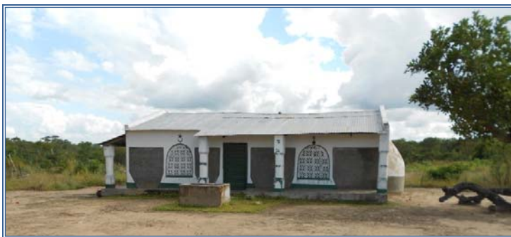
Figure 31: Mosque on the Mocubela-Bajone road
