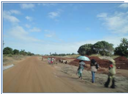
Figure 32: Local road use on Mocuba-Nipalaga road
