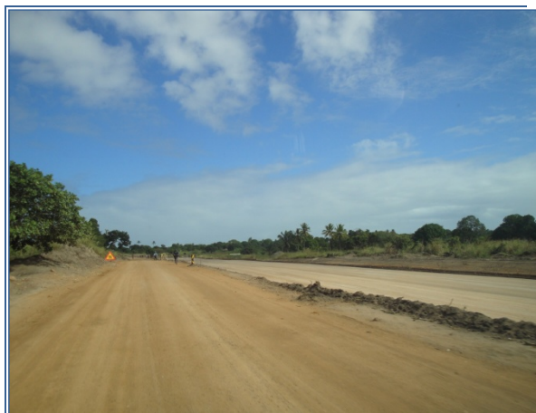
Figure 2: Road rehabilitation – pre-asphalt
