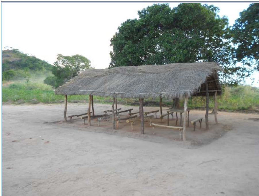
Figure 29: School on Mugulama-Ile road
