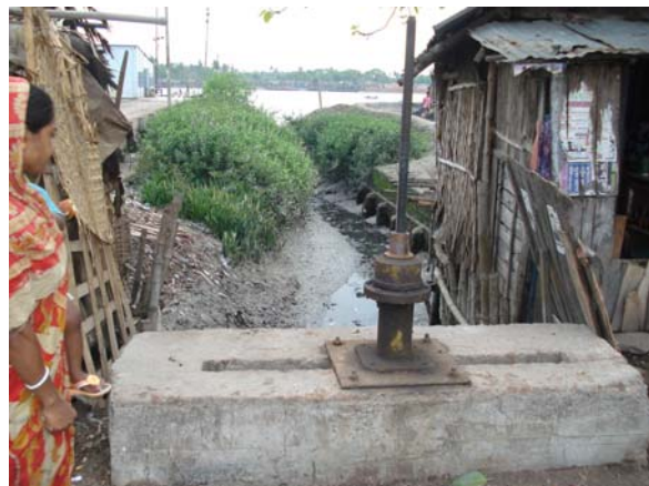
b. The sluiceway during low-tide
