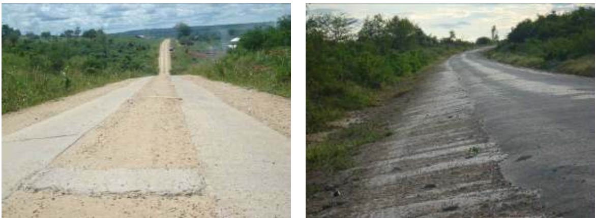
Figure 2: Concrete strips (left) and concrete geocells (right) as seen in Bagomoyo.
