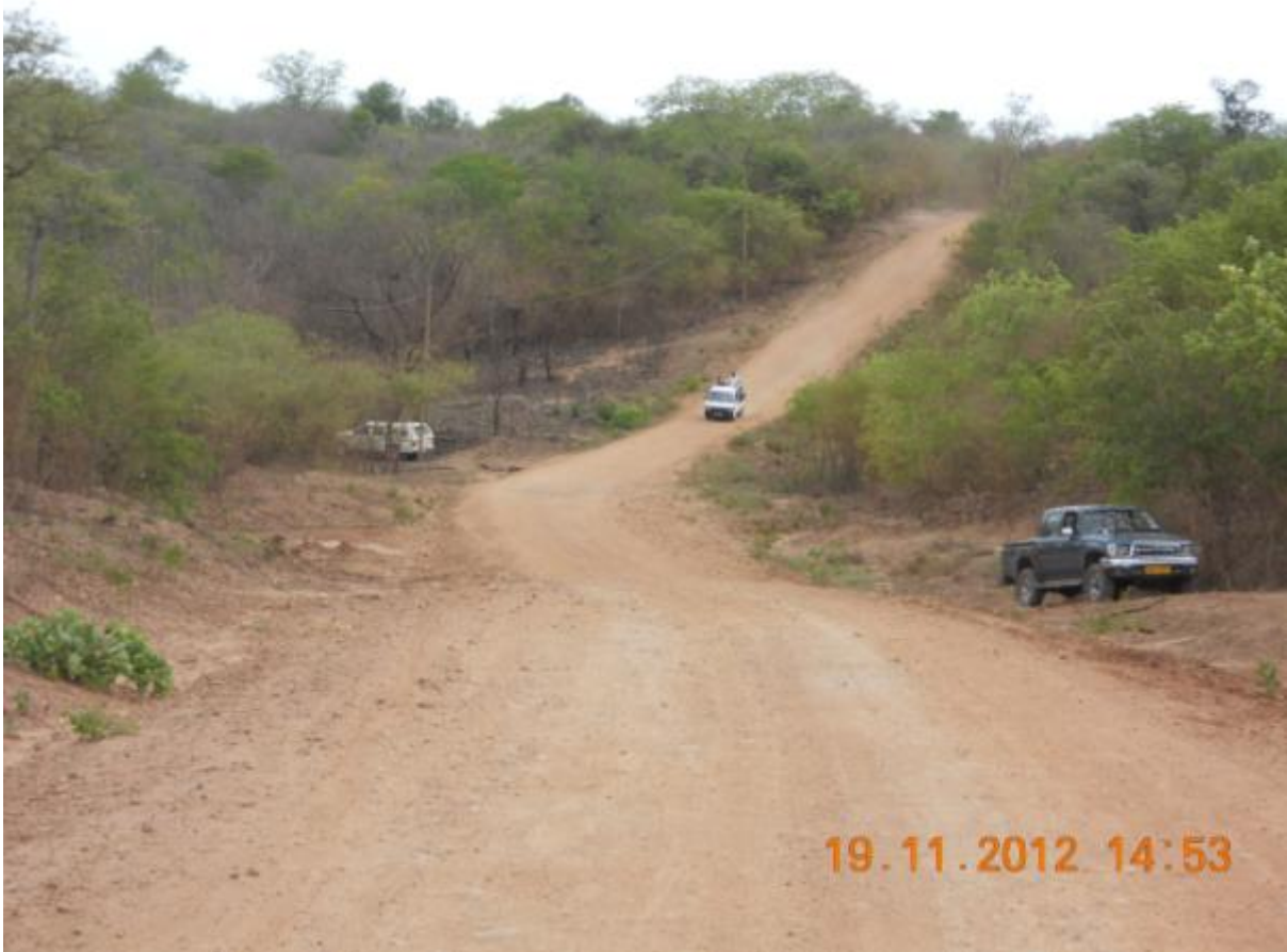
Photo 8: Guezanhe: Proposed Road Dam R521 crossing of Rio Tomere headwaters in a triple 800mm dia. culvert. Note the very good approach gradients for raising the embankment.
