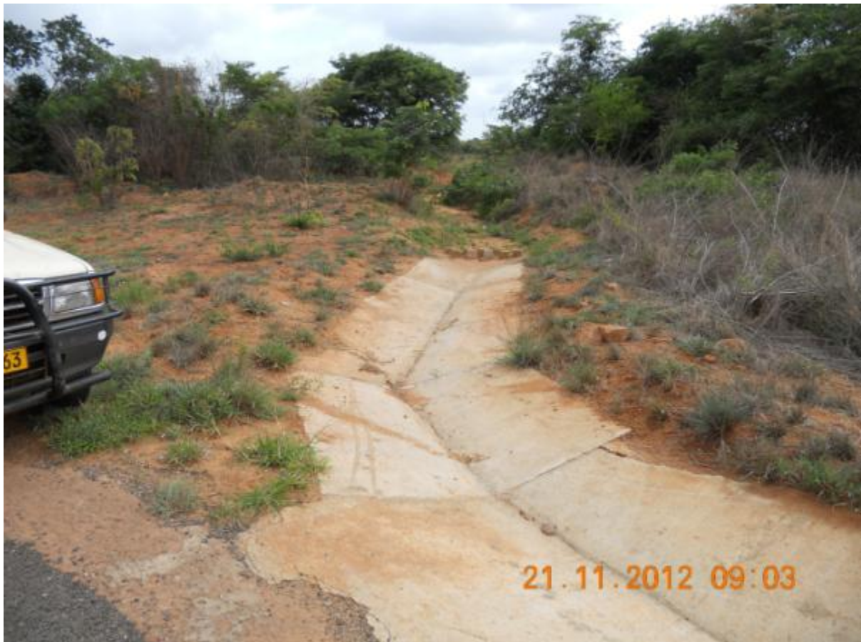
Photo 1: Nhambuica: Improved Borrow Pit: Lined side drain from the N1 can be diverted into the pit, which can be glimpsed in the background.
