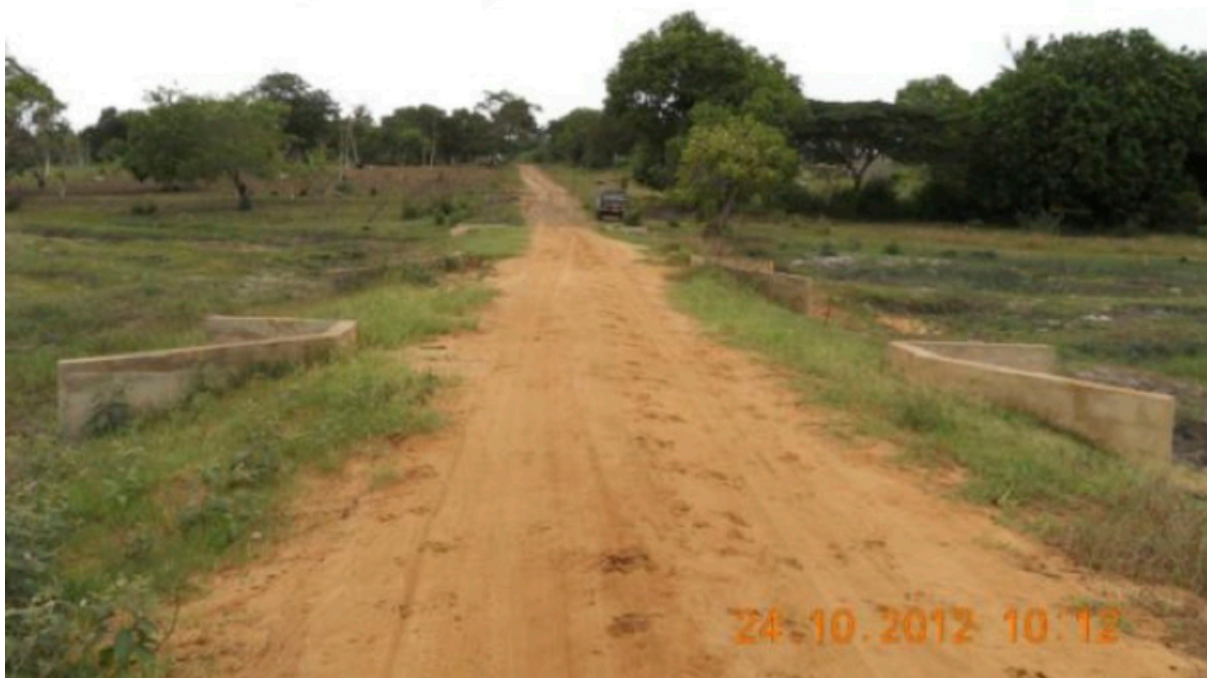
Photo 2: Tambajane: Proposed Road Dam: Existing embankment, incorporating three culverts, across the Rio Tendele drainage line is to be raised
