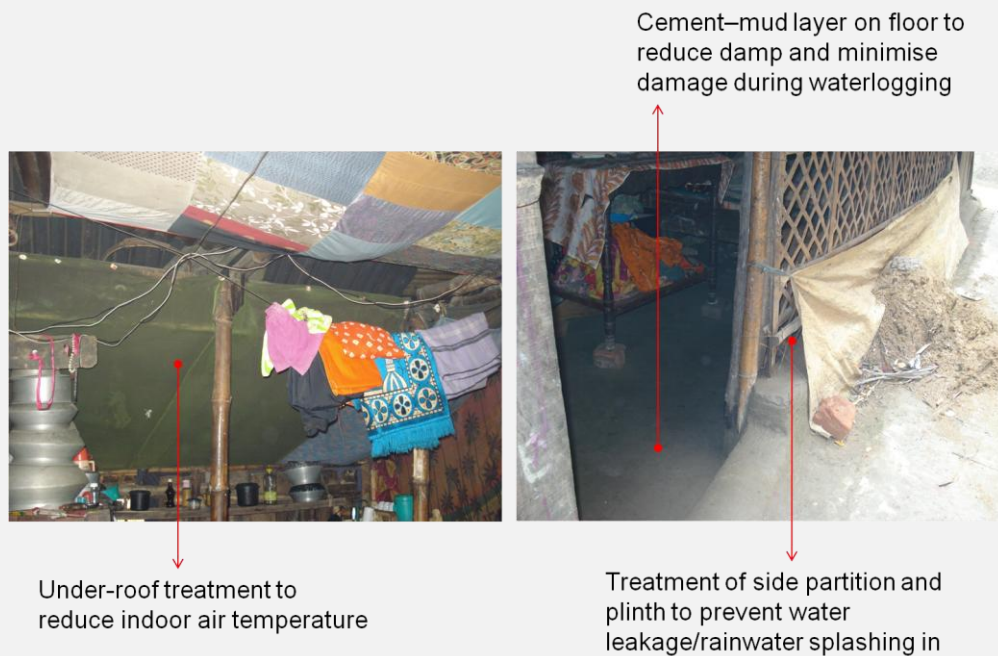
Figure b: Roof, floor and backside views of the dwelling
