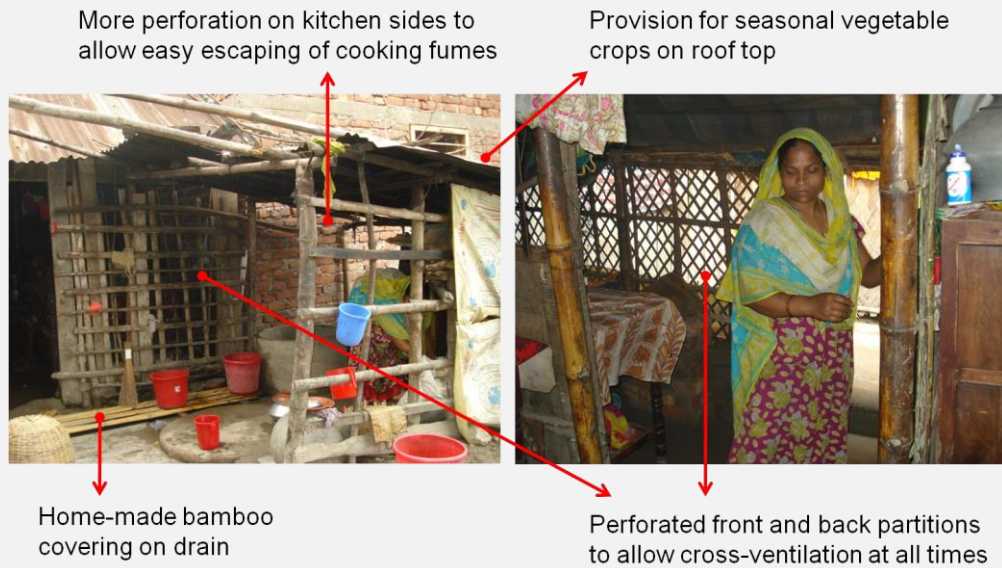
Figure a: Front and back side (seen from inside) of the dwelling
