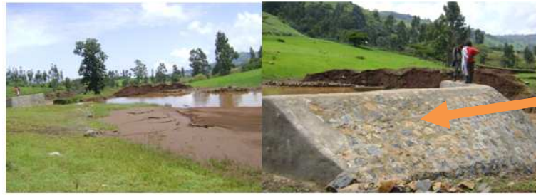
Figure 4 Sedimentation problems at Tulu Gurji kebele dam project at Mekja River
