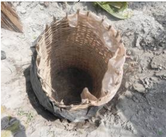
A low-cost latrine in construction, with polythene-lined bamboo cage already installed.
