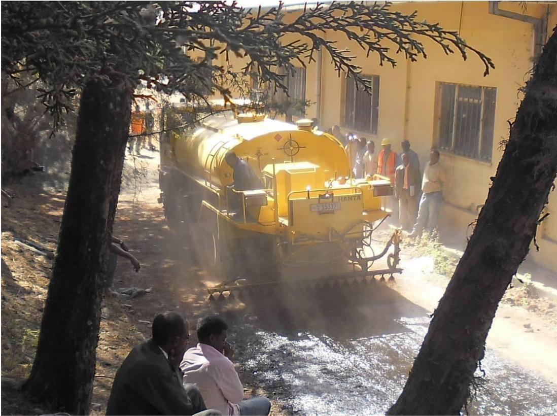
**Figure 4** Spraying MC 30 during the practical demonstration
