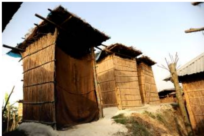
Low cost latrines raised above flood levels
