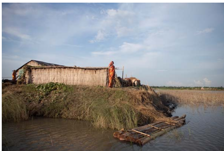
Earthen plinth raised above flood levels
