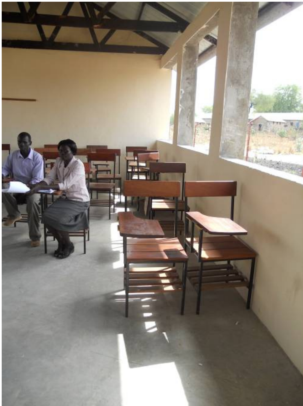
Plate 5 YEP classroom showing sun entering classroom in afternoon due to poor orientation
