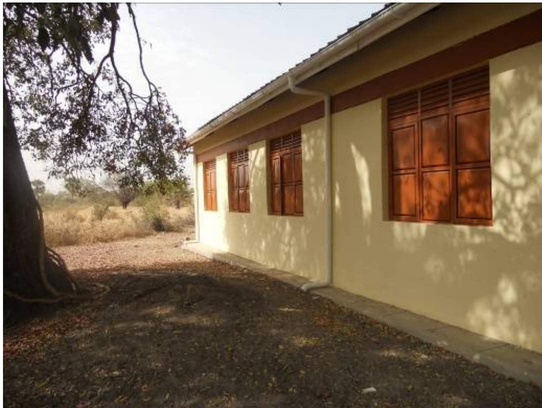
Plate 8 View of classroom building showing separate veranda roof and tree very close to building
