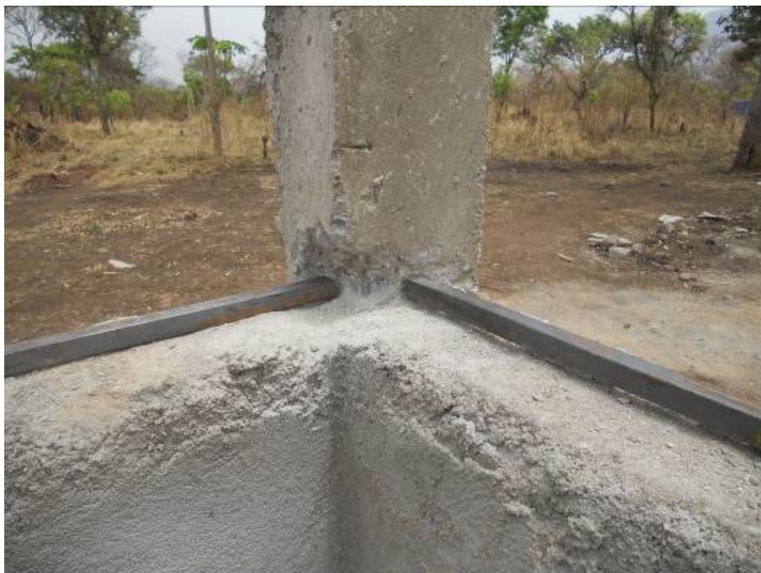
Plate 16 Columns to kitchen cut into at base for steel frames
