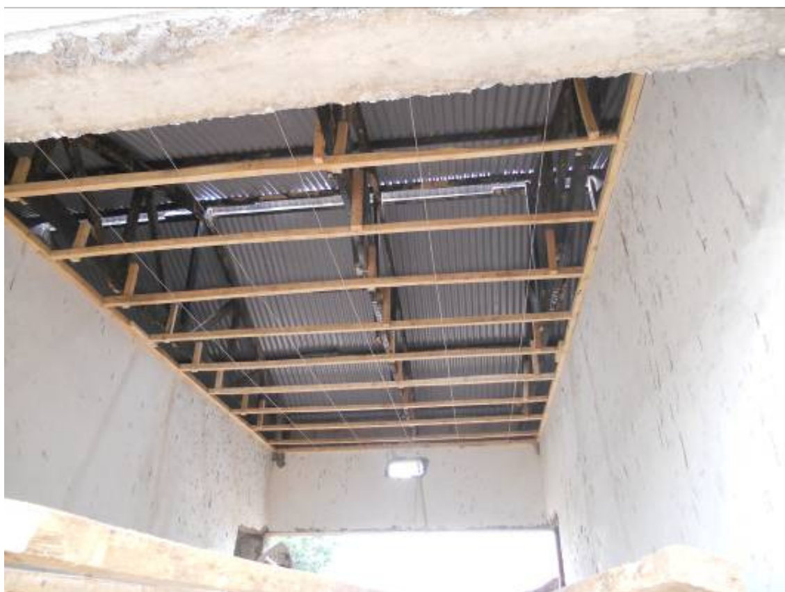
Plate 14 Badly built cross walls and inadequately treated roof timbers
