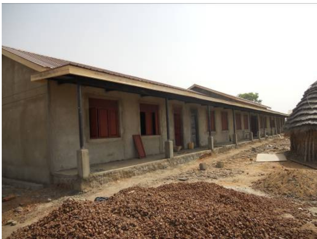
Plate 10 View of administration/classroom building showing almost flat veranda roof
