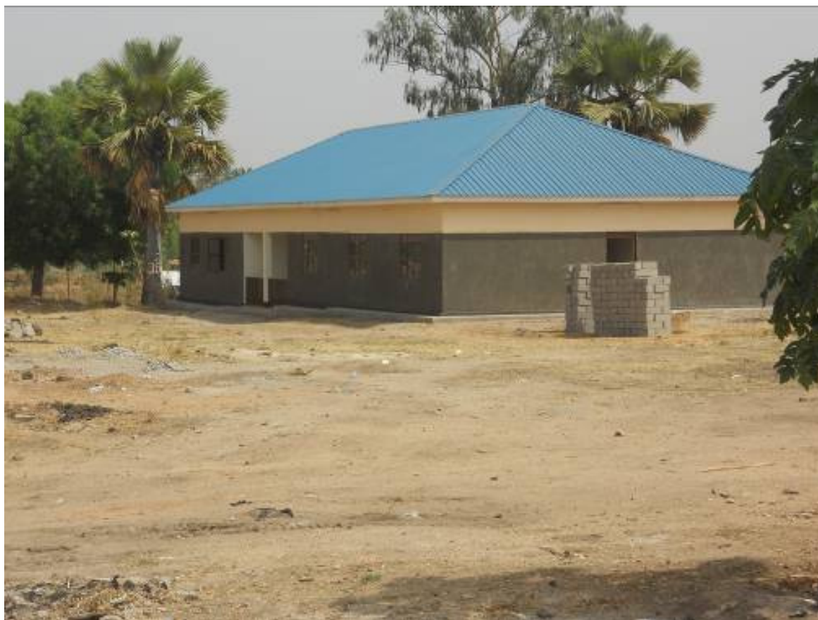
Plate 6 Dormitory showing lack of windows and poor design
