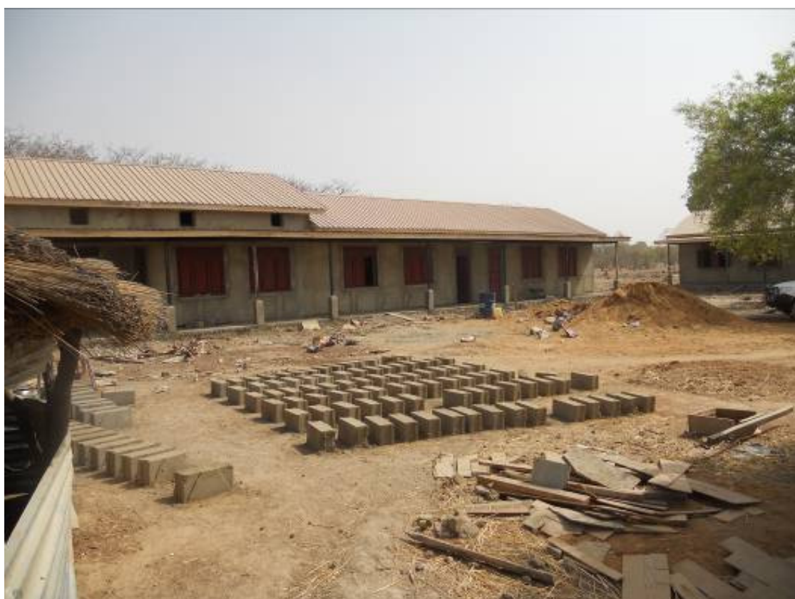
Plate 12 More blocks drying too quickly under the sun
