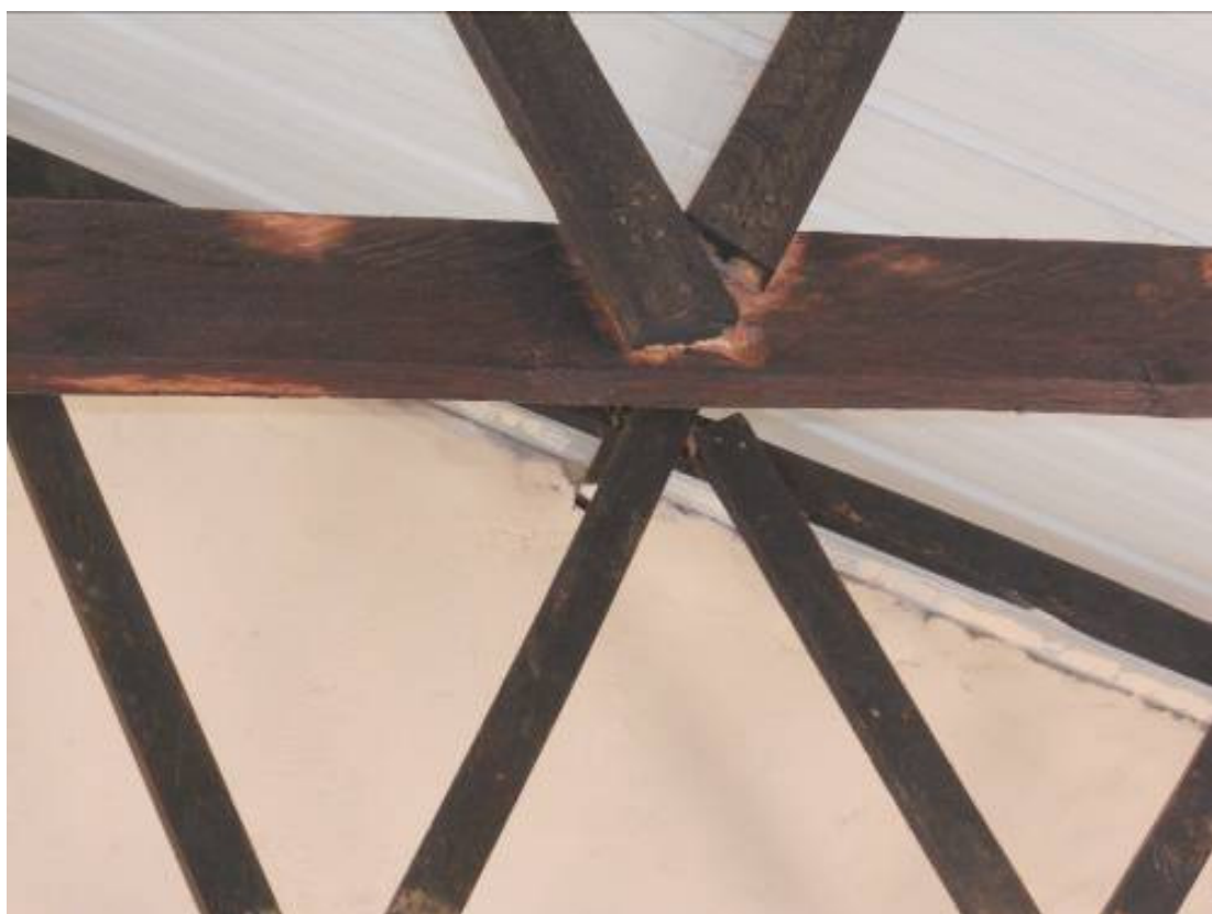
Plate 3 Typical roof truss showing very badly made joints
