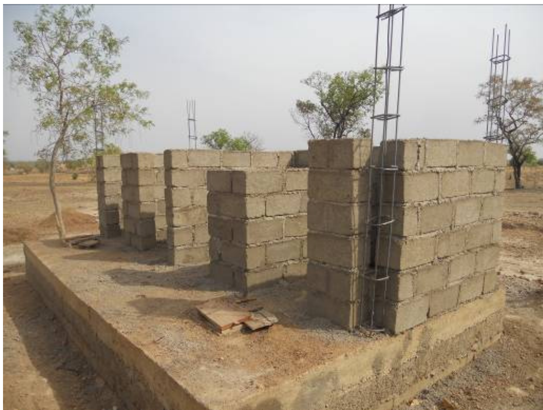
Plate 2 Blocks being made in the open with no cover and no chance therefore of being properly cured
