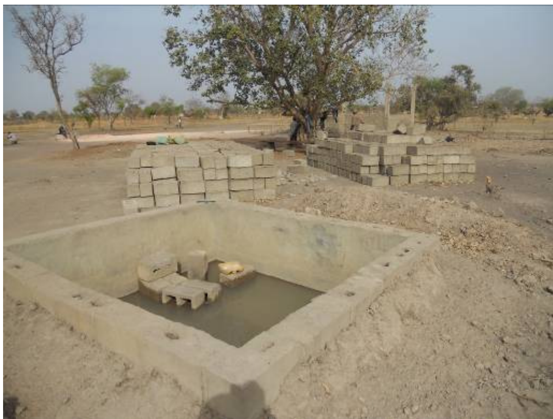
Plate 2 Blocks being made in the open with no cover and no chance therefore of being properly cured
