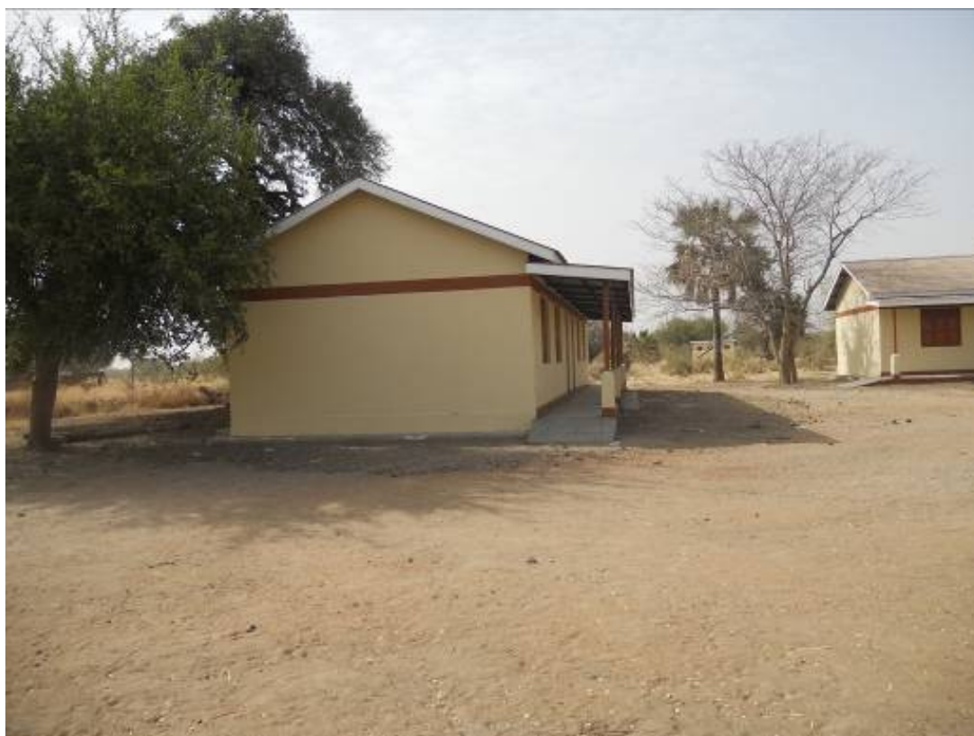
Plate 8 View of classroom building showing separate veranda roof and tree very close to building
