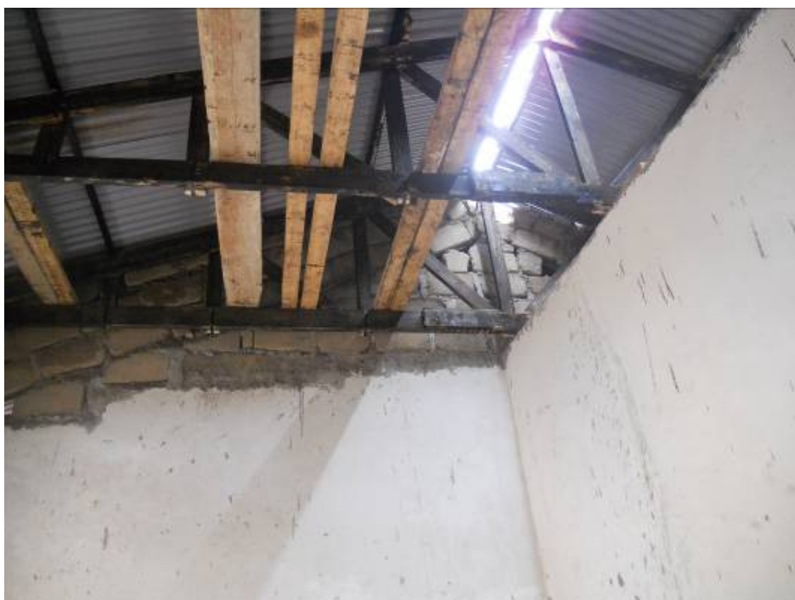
Plate 14 Badly built cross walls and inadequately treated roof timbers
