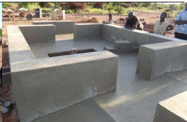
**Figure 7: Accessible handpump apron, Moribila Zounoukan. Seating block is visible**
