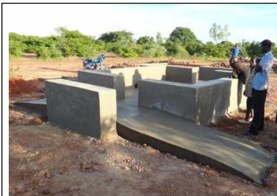
**Figure 6: Accessible handpump apron, Moribila Ziékan, showing access ramp**
