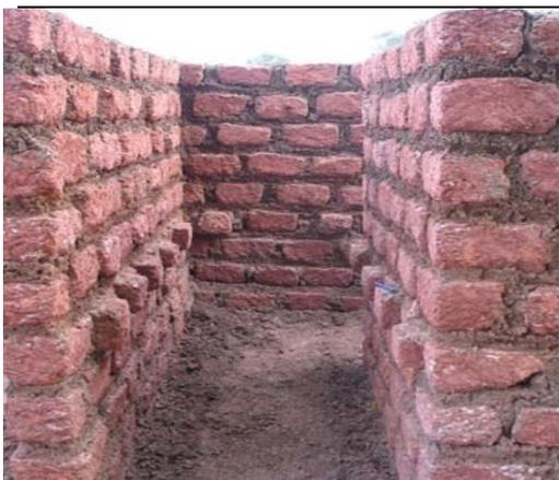
**Figure 18: Protruding bricks for support to enter/exit a latrine**
