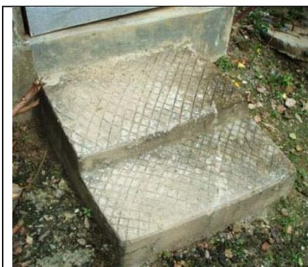
**Figure 24: Low steps with cross-hatching**
