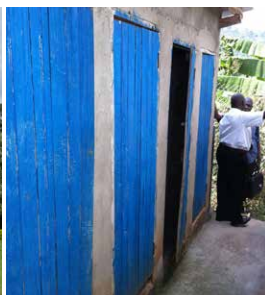
Cramped water closets
