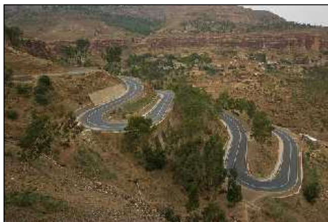
Typical Hairpin bend stack on main road between Adigrat and Enticchio.
