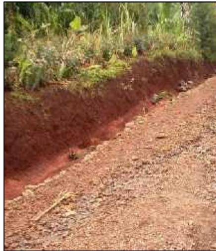
Gravelled shoulders. (Note the larger stones retaining the gravel edge)
