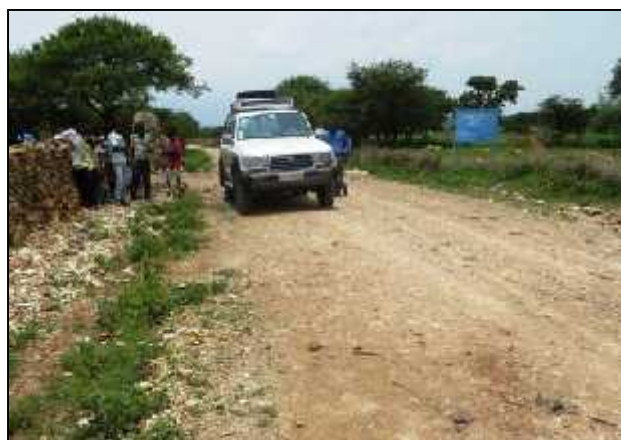
An Example of a URRAP road constructed with a relatively high degree of community contribution. (Note: no side ditch and no camber. The contractor's contract was for gravelling only.)
