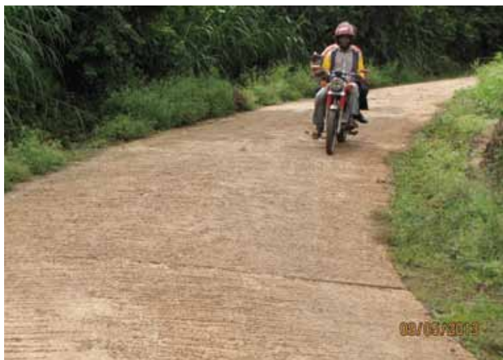
Photo 7-5: Example of reinforced concrete surfacing
