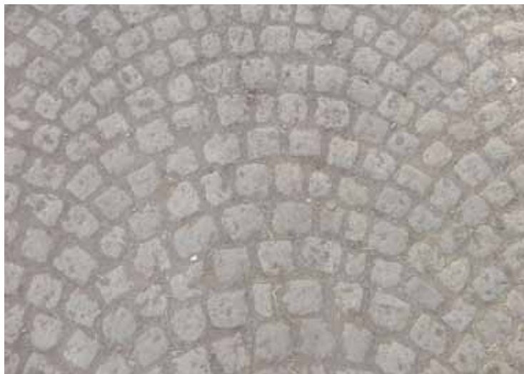
Photo 7-1: Example of Cobble Stone surfacing
