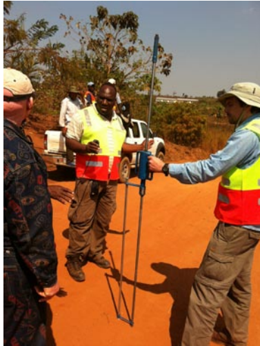
DCP test demonstration by Aurecon team
