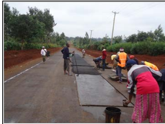
Figure 3: Spreading and levelling CMA between guide rails
