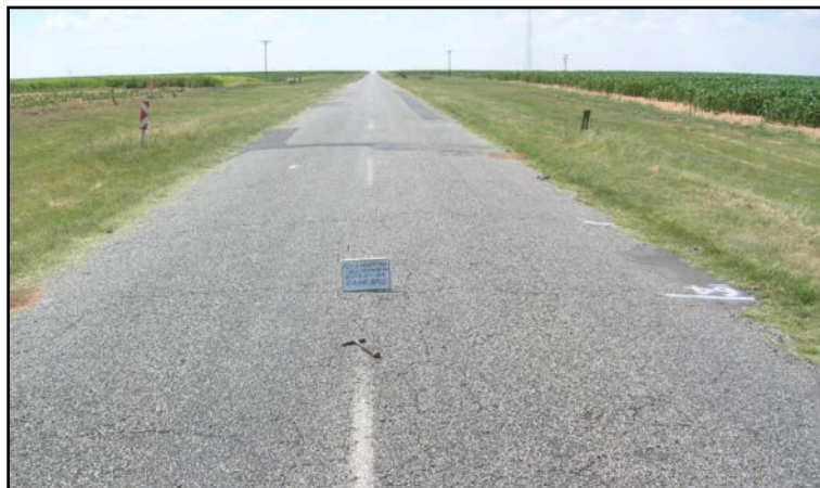
Figure 1: Hoopstad-Bultfontein Experimental Section (South Africa) built in 1962 with neat sand base
