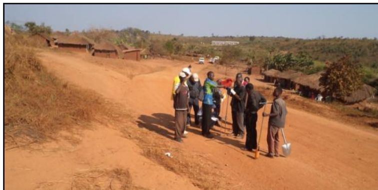
Figure 6: DCP testing in DRC
