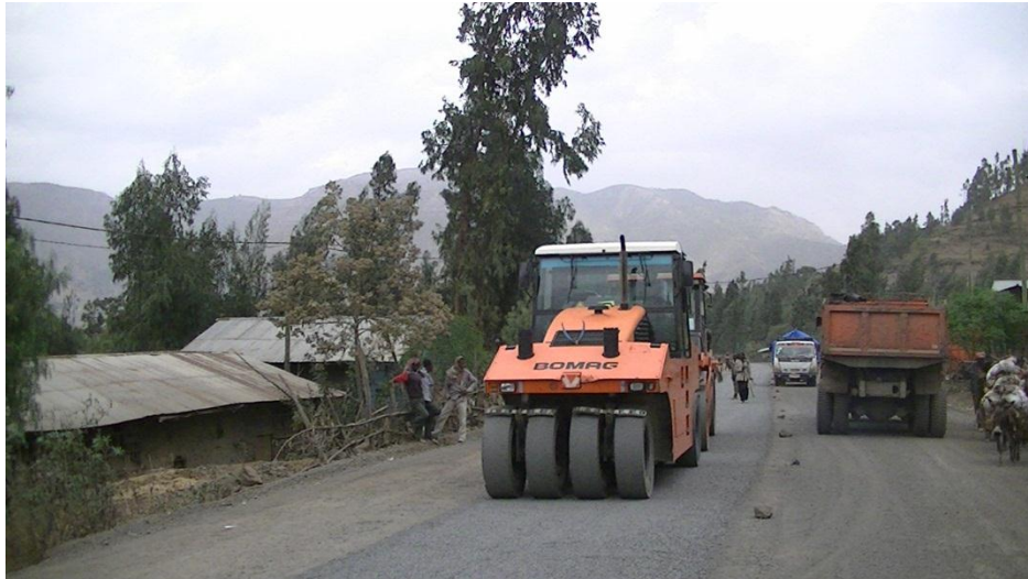
Figure 4-4 Rolling in progress by the use of both a pneumatic roller and the loaded tipper truck
