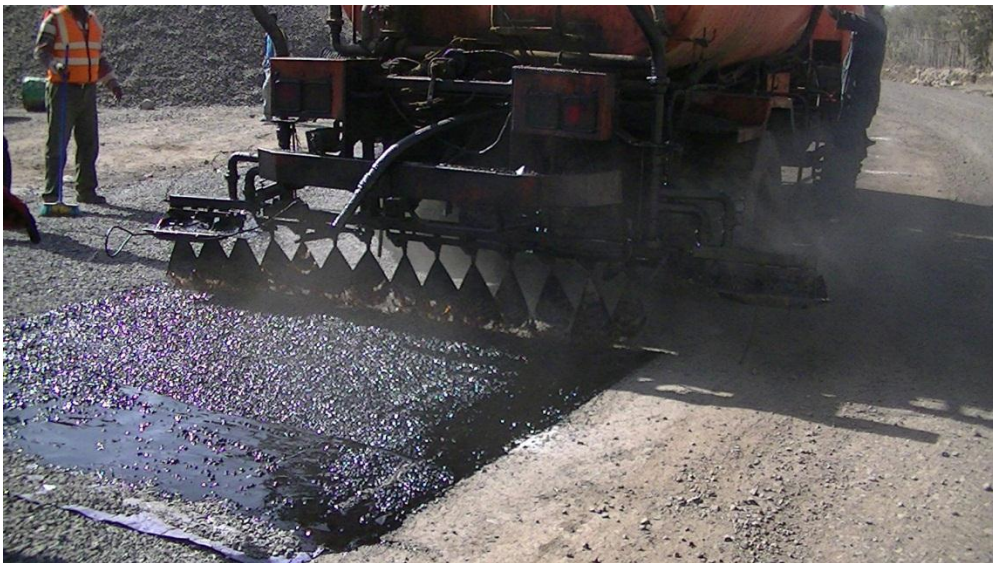
Figure 4-2 Paper used to achieve straight transverse joints
