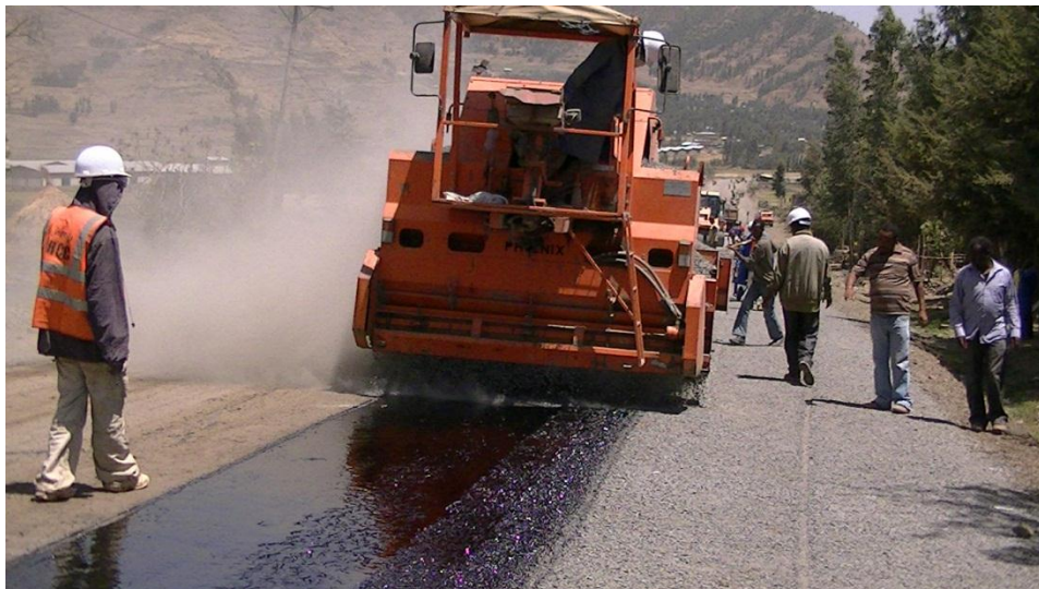
Figure 4-3 Self-propelled chipspreader in operation
