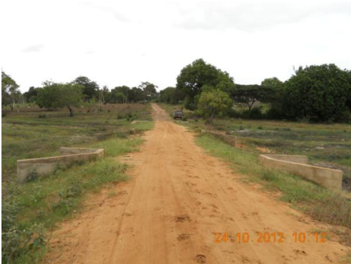
Photo 2: Tambajane: Site of Proposed Road Dam: Existing embankment, incorporating three culverts, across the Rio Tendele drainage line
