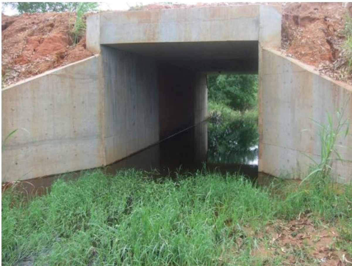
Photo 3: Inhamussua: Site of Proposed Road Dam An existing box culvert in high embankment can form a road dam without raising
