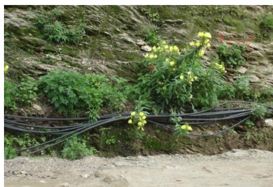
Individual hosepipe connections to the source
