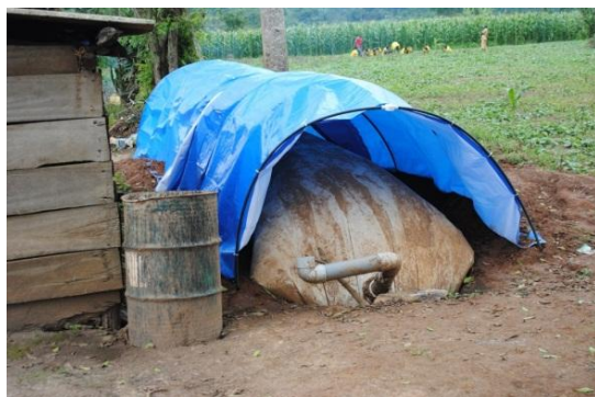
Figure 2.5.12 - Plastic sheet shelter
