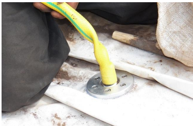
Figure 2.5.5 - Hose tube on a gas connector
