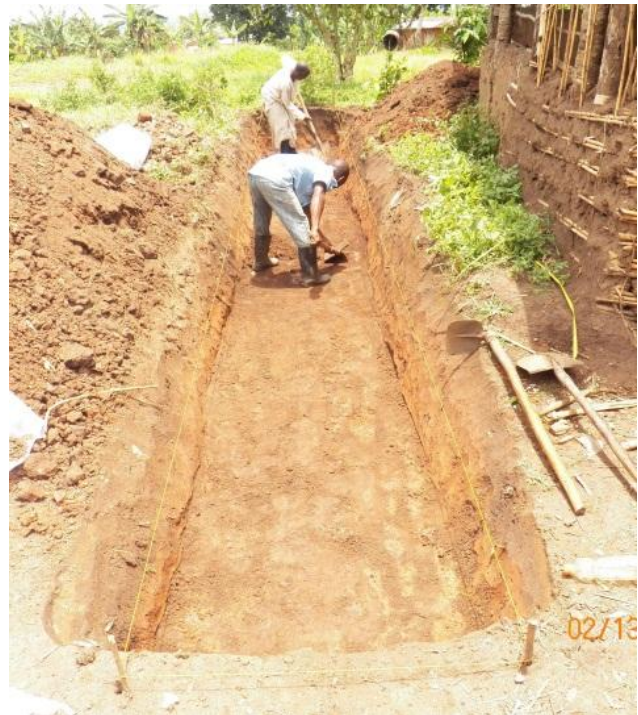
Figure 2.5.2 – Shaping of the sides of the ditch
