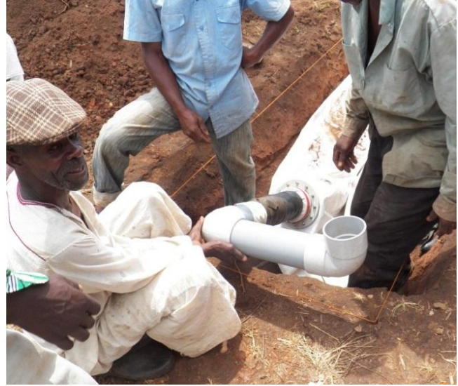
Figure 2.5.4 - Inlet pipe
