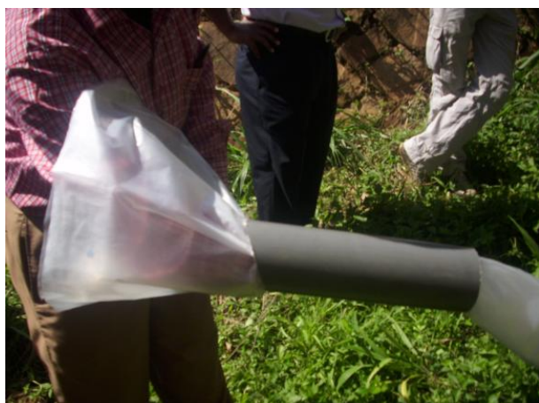
Figure 9.2.2 – Attaching the inlet and outlet to the folded plastic digester
