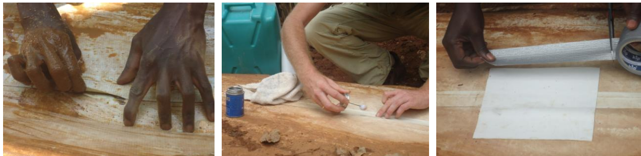
Figure 2.4.6 – Fixing faults: (a) Un-welded point on a digester (b) Glue applied to fix the digester (c) Taping the glued section
