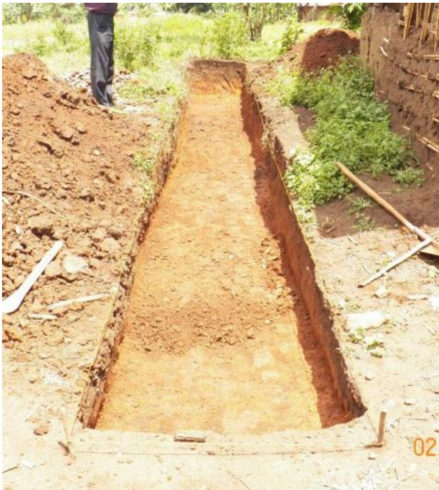
Figure 2.5.1 - Ditch with vertical walls
