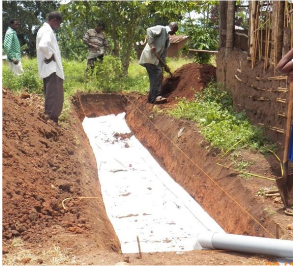
Figure 2.5.3 - Digester in the ditch
