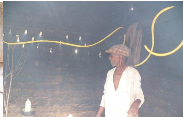
Figure 2.5.6 - Gas pipe into the kitchen
