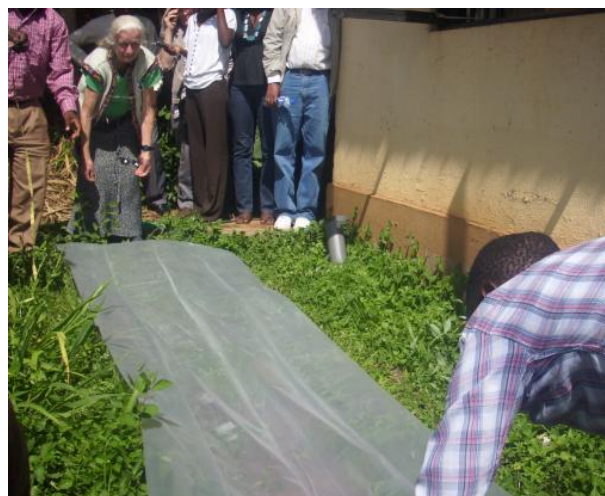
Figure 9.2.1 – Laying out the plastic tube, ready to construct a folded plastic digester
