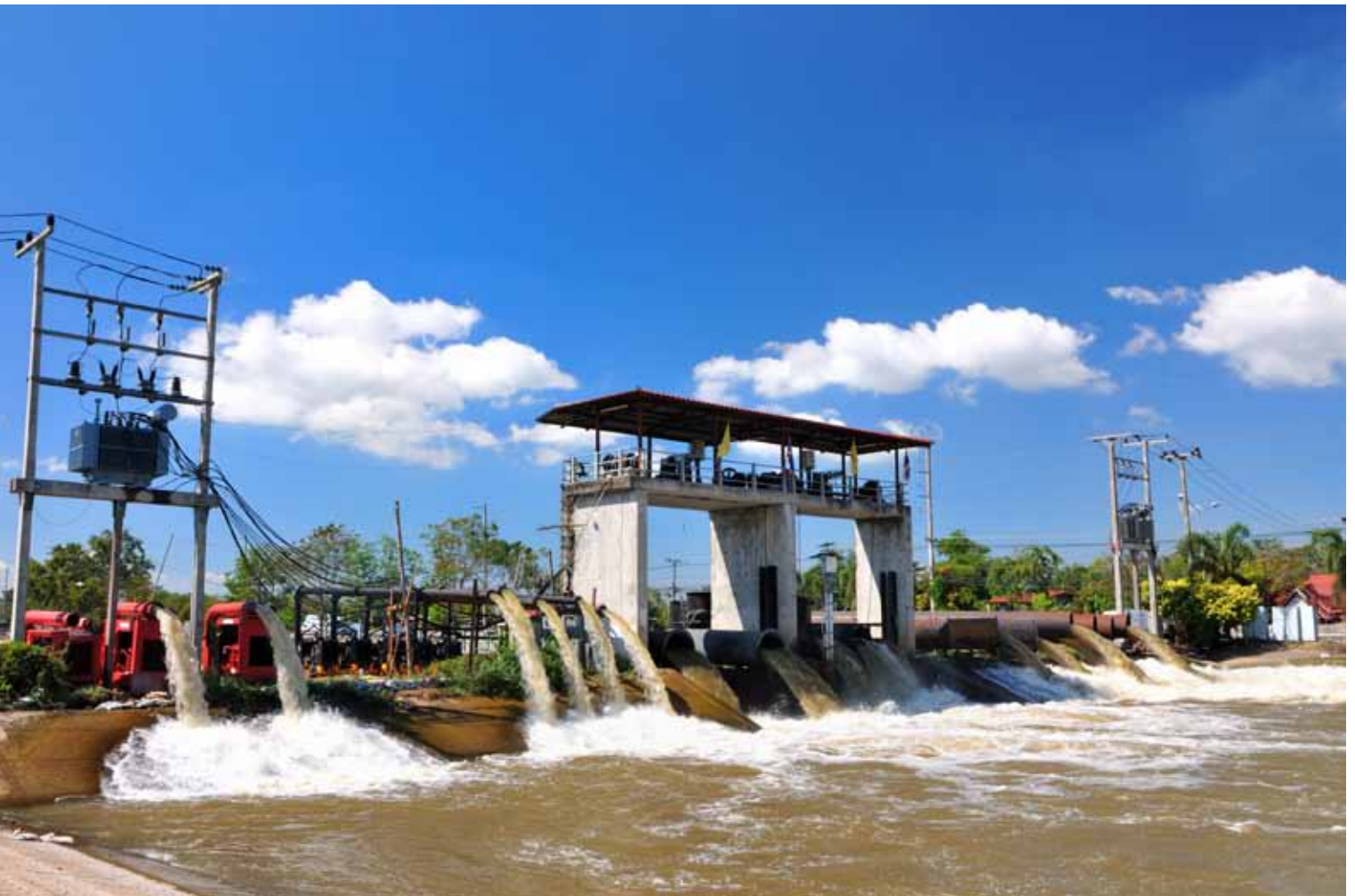
Floodgate opening to release flood waters
