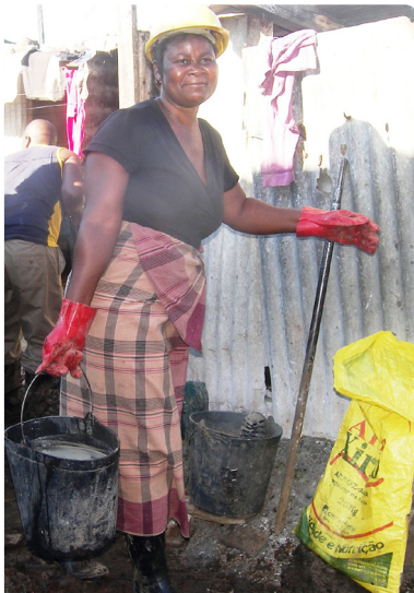
Women-led construction in Maputo, Mozambique
