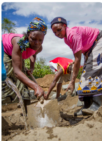
Women working in latrine construction in Naivasha, Kenya
