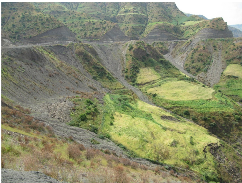
Figure 9: Large quantities of sediment generated by spoil disposal and erosion below roads
