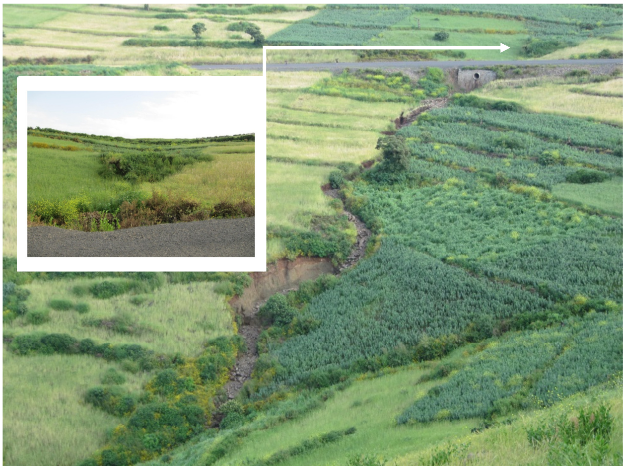
Figure 7: Erosion beneath culvert outlet due purely to road runoff (note lack of stream channel above the road)
