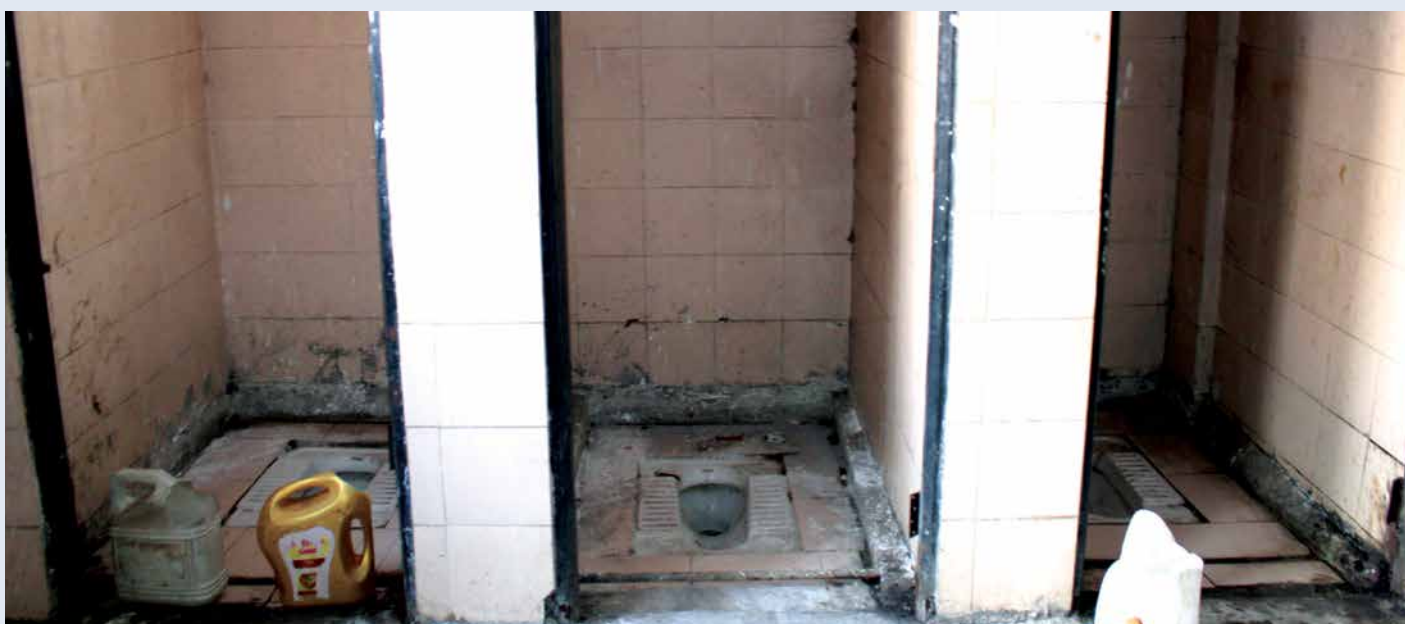
Pit toilets without doors, Pune. Photo credit: Lakshmi Anantnarayan
