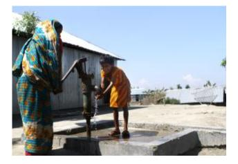
Where tube wells exist and meet certain criteria, CLP upgrades them by installing a concrete platform. This prevents groundwater contamination through the base of the well.
