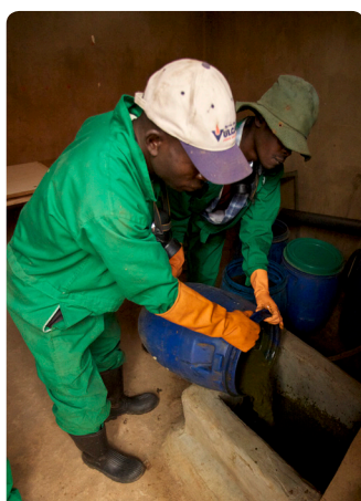
Pit-emptiers tip sludge into the holding tank of a public toilet
