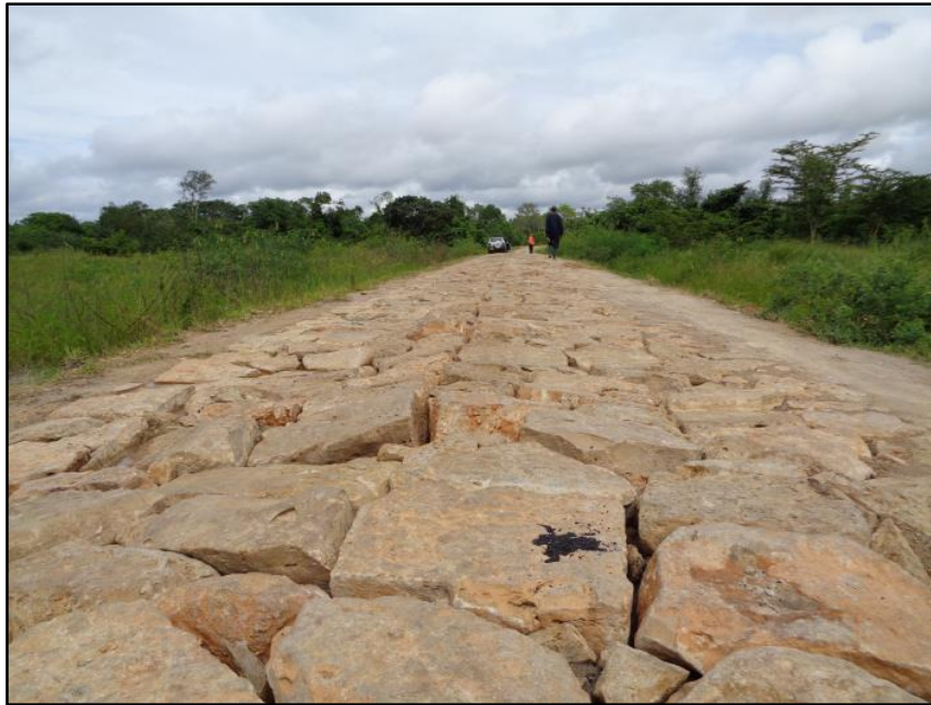
Photo 13: Rough Hand-Packed Stone Blocks (B-T)
