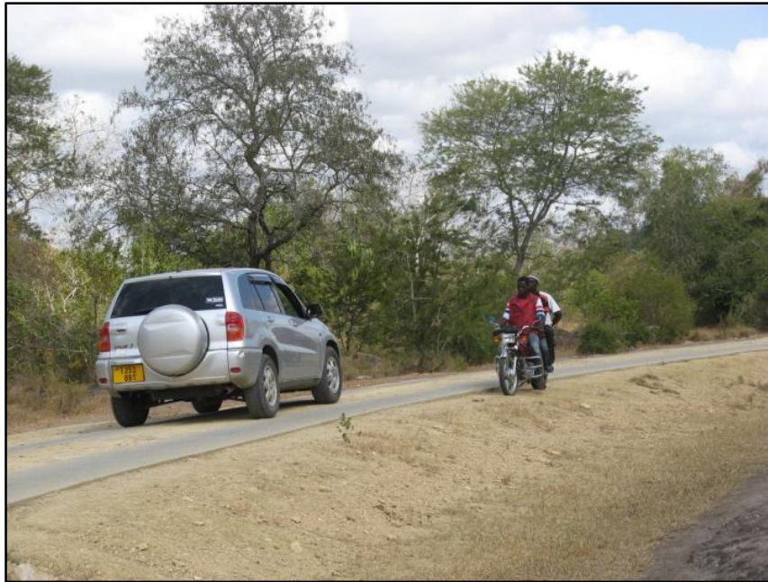
Photo 10: Absence of Adequate Shoulder with Parallel Concrete Strips (B-T)
