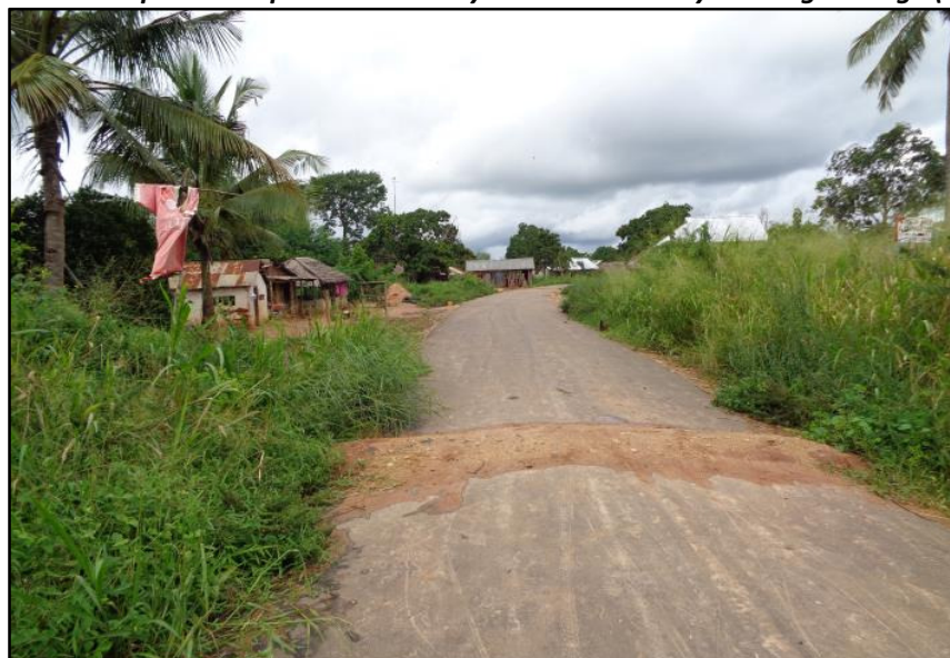
Photo 18: A Speed Hump Constructed By Local Community in Ludiga Village (B-T)
