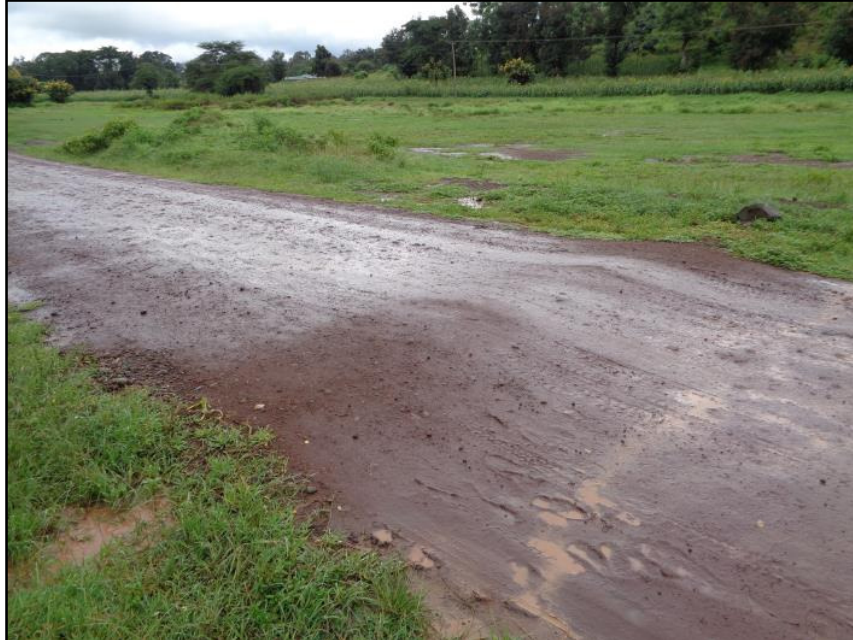
Photo 19: An Earth Speed Hump Constructed By the Siha District Engineer (L-K)
