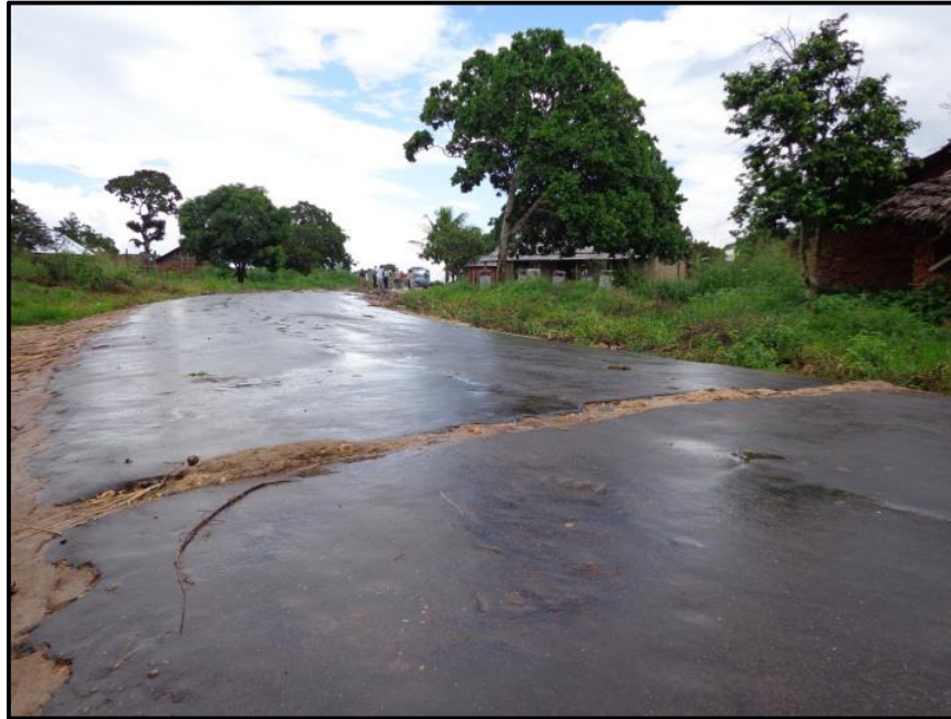
Photo 4: Smooth and Wet Double Sand Seal Surface (B-T)
