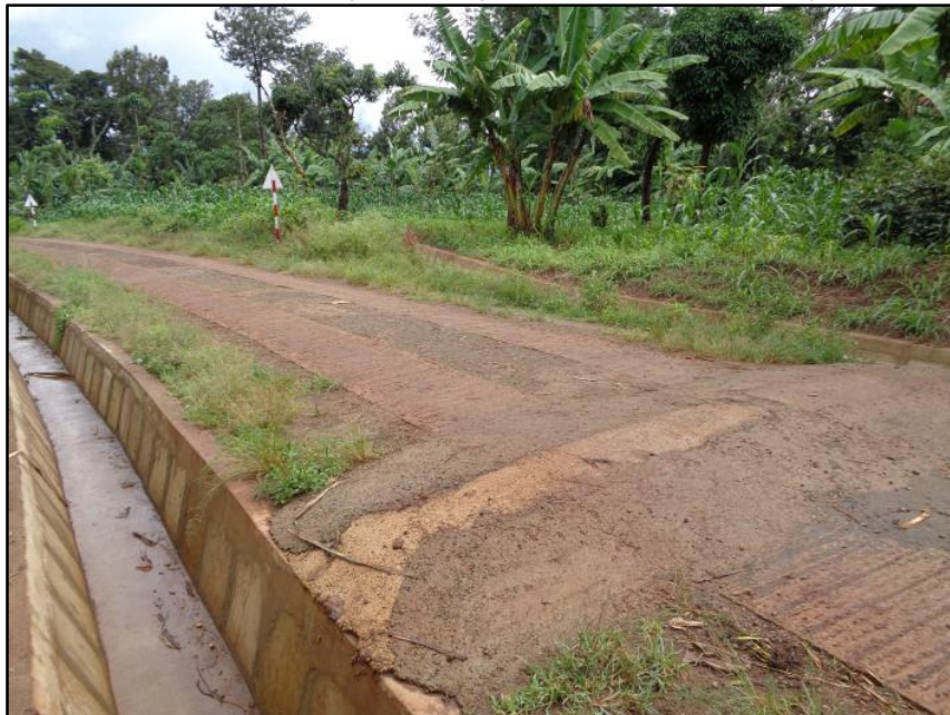
Photo 20: A Concrete Speed Hump on Parallel Concrete Strips (L-K)
