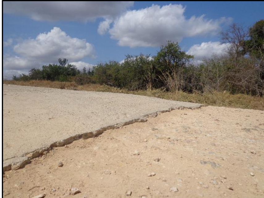
Photo 8: Un-level Join between Surface Types (B-T)
