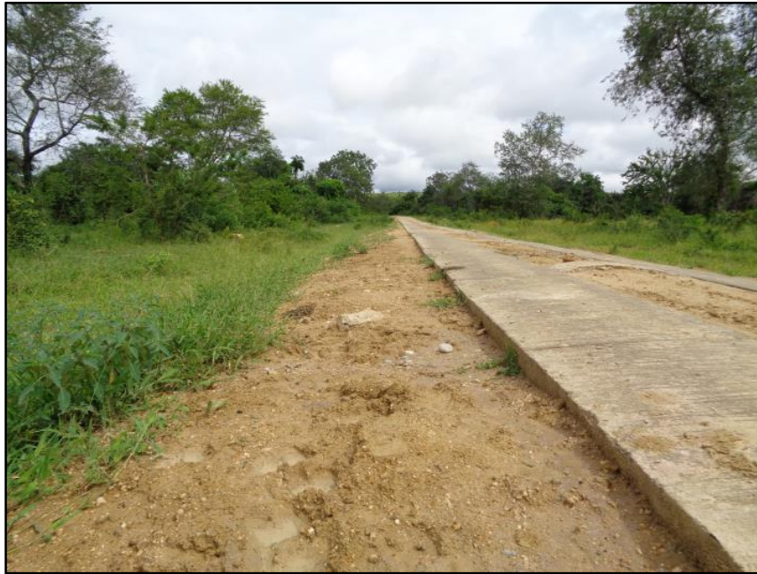
Photo 10: Absence of Adequate Shoulder with Parallel Concrete Strips (B-T)
