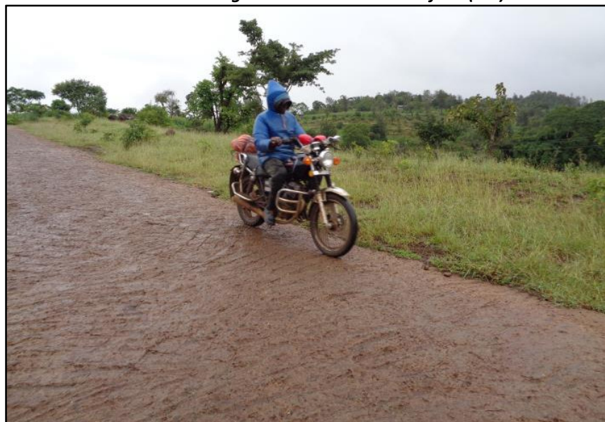
Photo 6: A Rough Concrete Geocells Surface (L-K)
