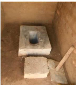
**Rammed earth floor made of marram (small stones) and sand; cow dung is smeared over to make it even and smooth.**
