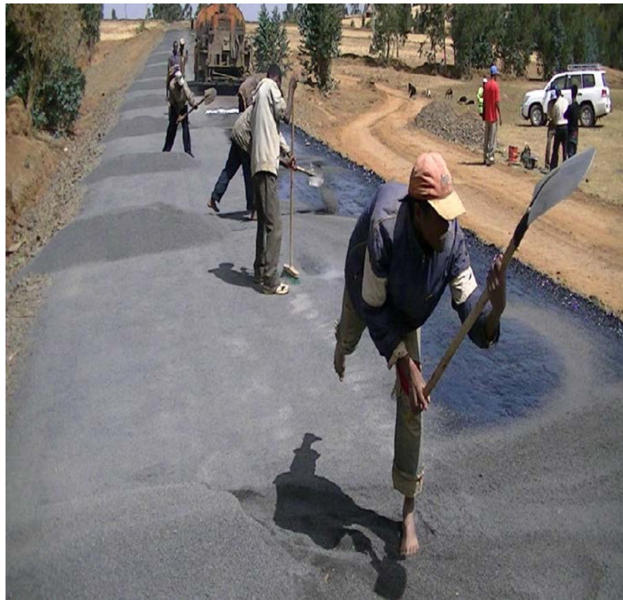
Application of crusher sand by labor
