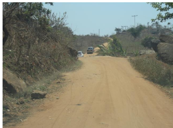
Picture 10: Section with blind curves and sharp crest that needs fully engineered solution
