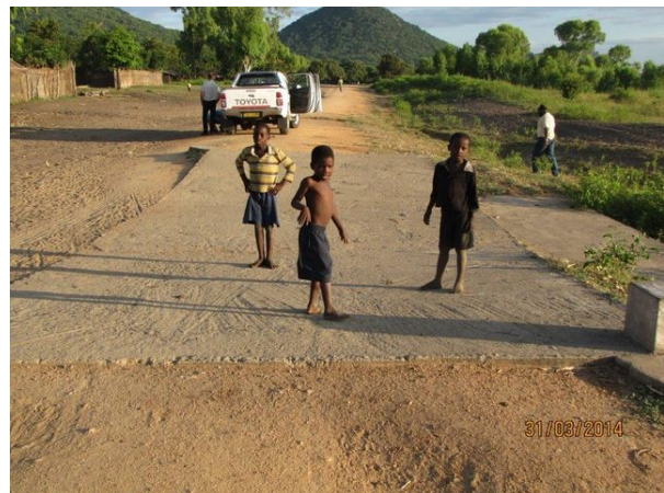
Picture 12: Non-functional drift in village on sandy sections
