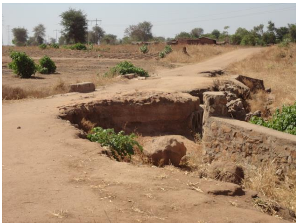
Picture 5: Erosion around existing drift
