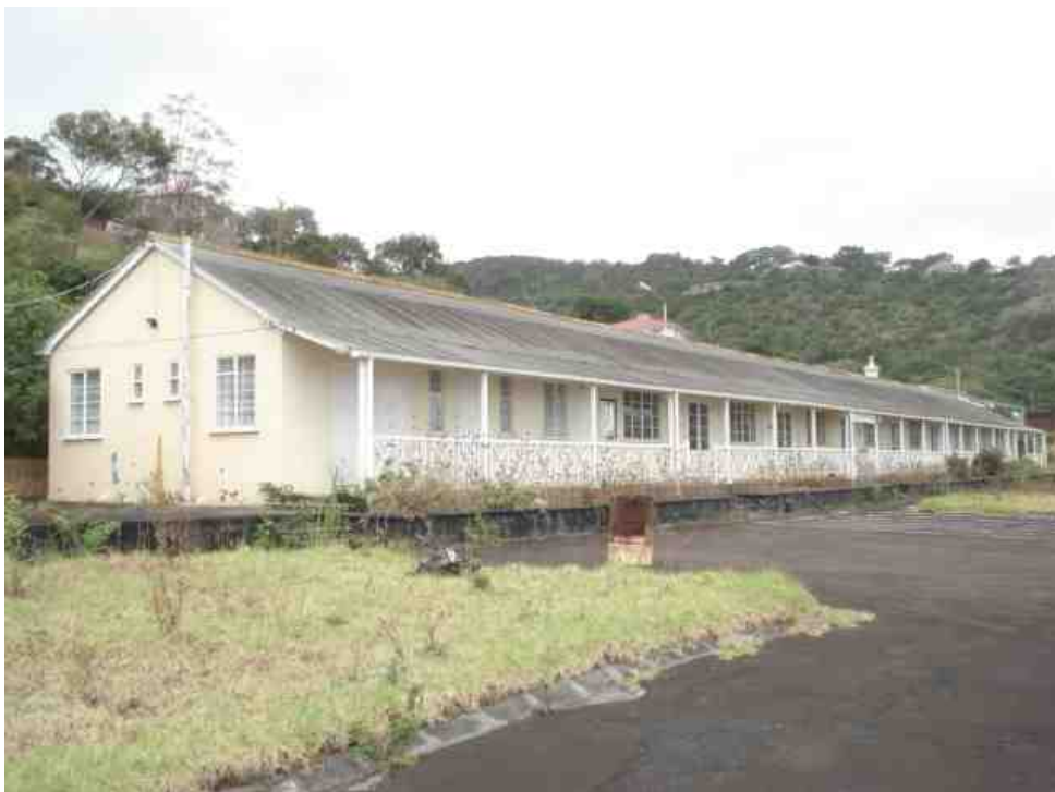
Figure 2: Main School building as existing
