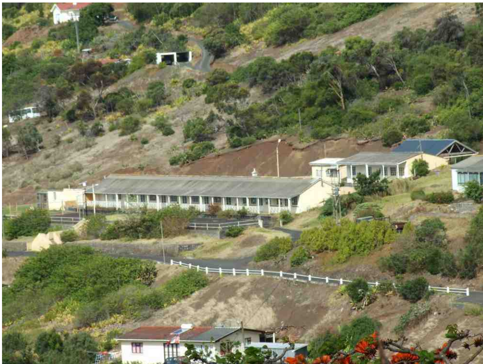
Figure 4: Long range front view of School
