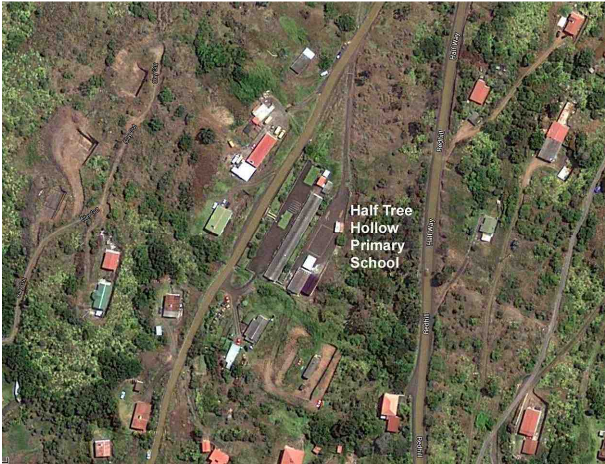
Figure 1: Aerial view of former Half Tree Hollow Primary School
