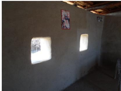
**Acceptability** – The shelter had good thermal mass with multiple openings resulting in good internal environment which was light and ventilated. However it was scored down on security as no windows or doors were provided. The shelter programme was integrated and no consideration was made for cooking and WATSAN.
