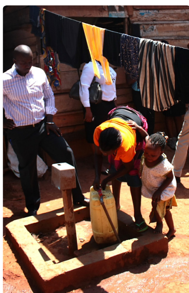
Group connection with metered standpost provided by NWSC, Kampala
