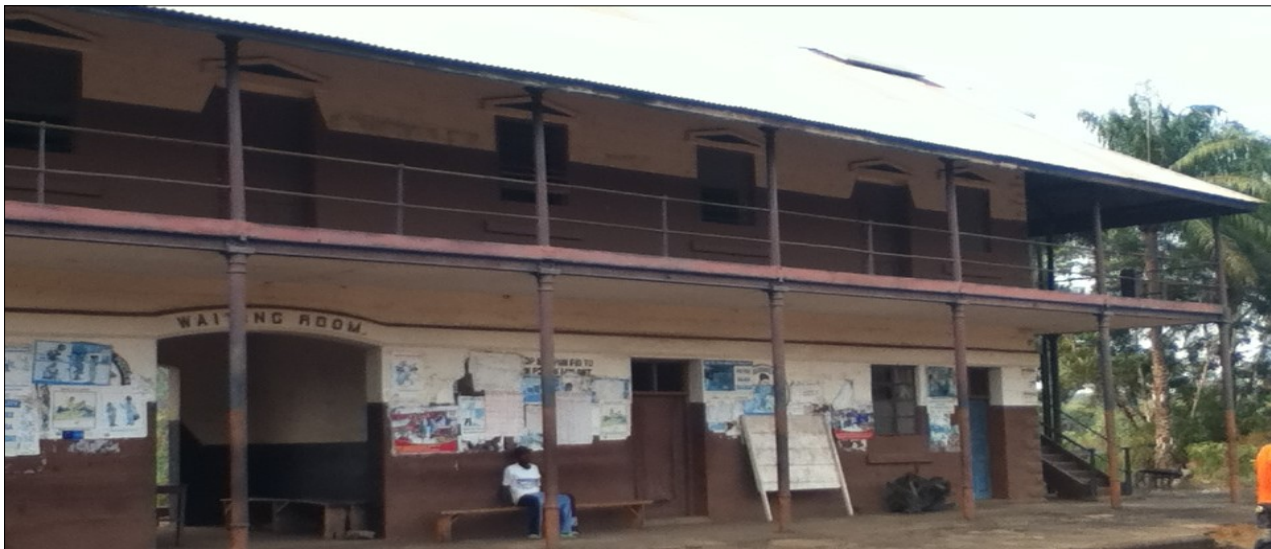
Health centre in Moyamba in the old train station (Photo: MP Bertone)
