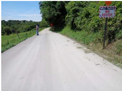
Shale gas well access road
